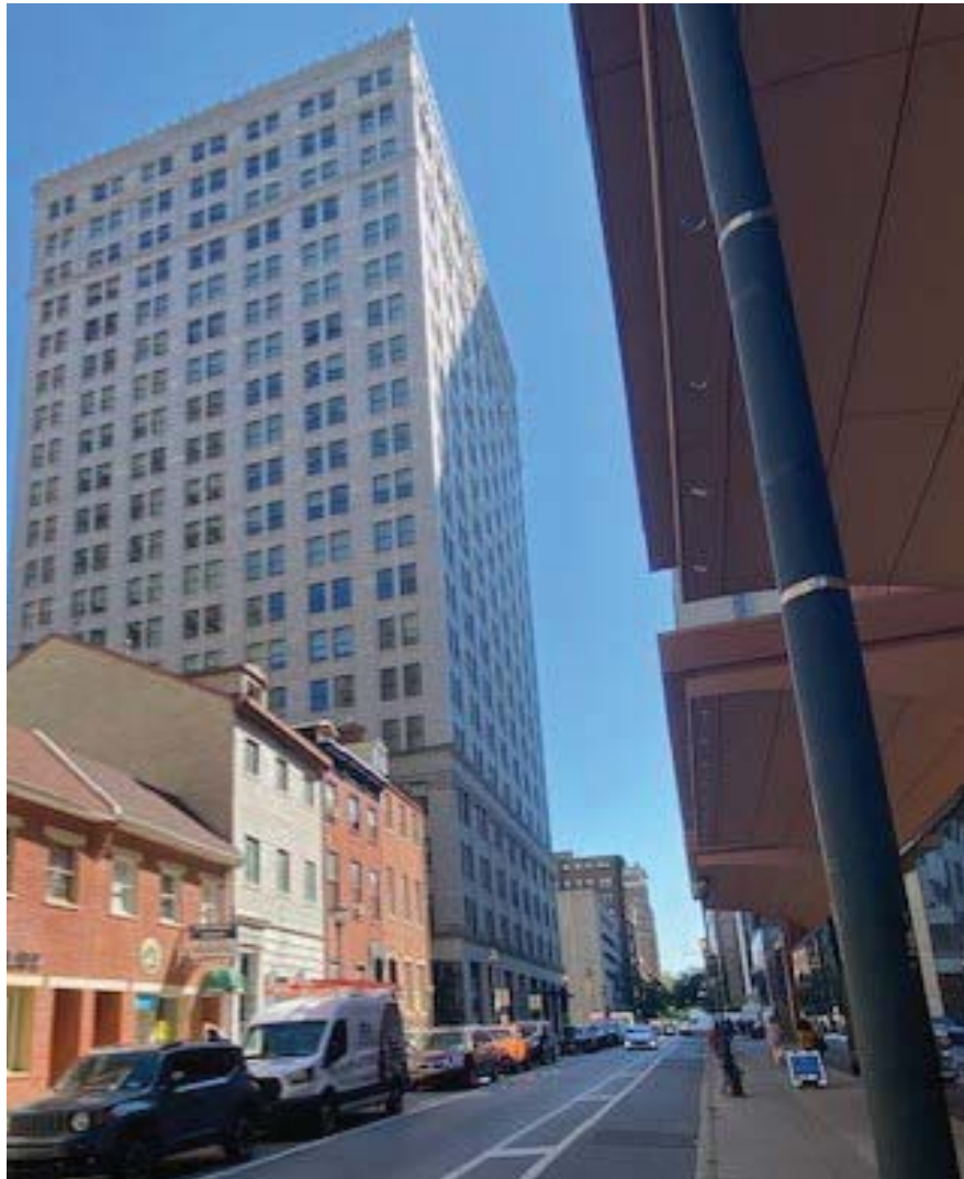
Figure 3. Spruce Street east of proposed building.
