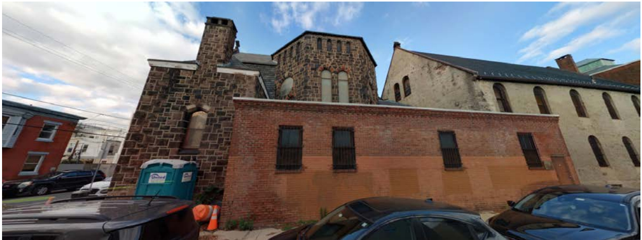
Figure 7. Rear (Montrose Street) elevation of church, showing one-story non-historic brick addition to be removed.
