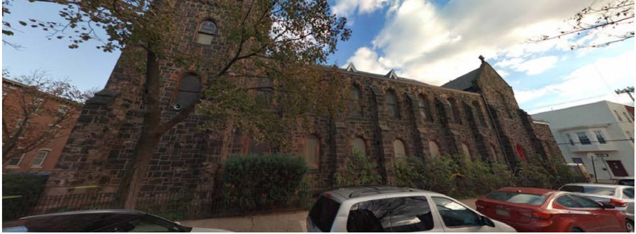
Figure 6. Side (21 st Street) elevation of church building.
