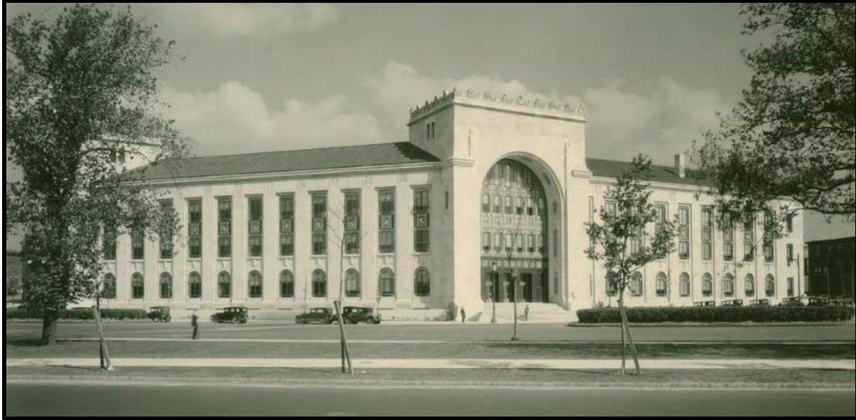
Figure 19. Fidelity Mutual Life Insurance Company Building, 1926, Zantsinger, Borie, & Medary, 26 th and Fairmount Avenue. Source: Building a Nation: Limestone Photograph Collection, Indiana University Bloomington.
