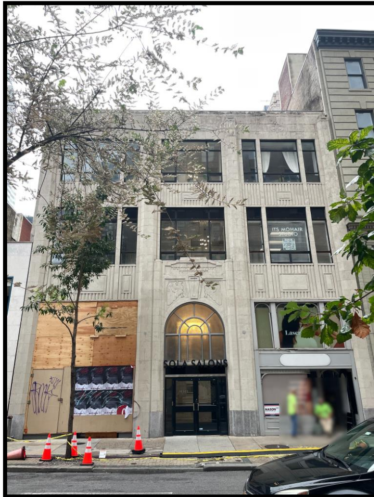
Figure 1. The primary (south) elevation of the subject property. Source: Ted Maust, 2023.
