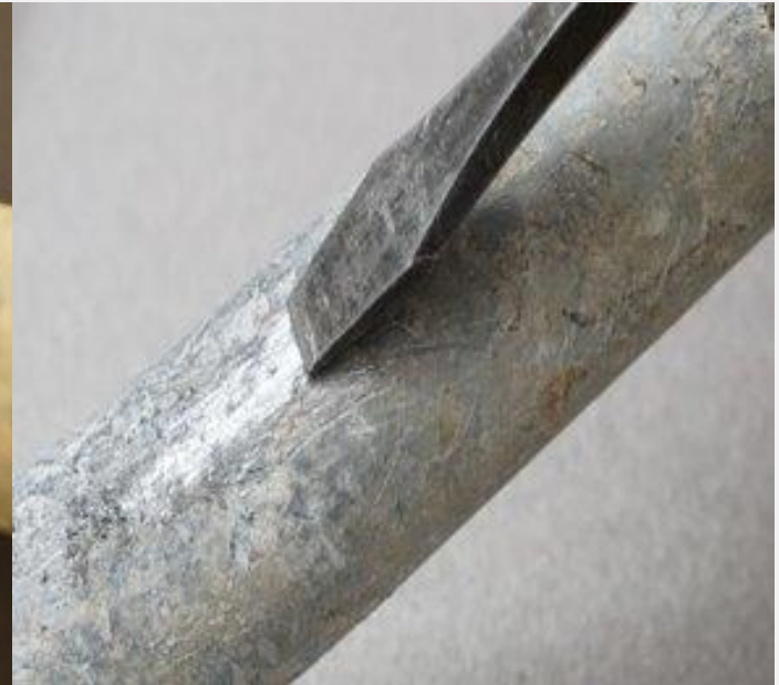
Lead Pipe Test: Scratch, and use magnet.
