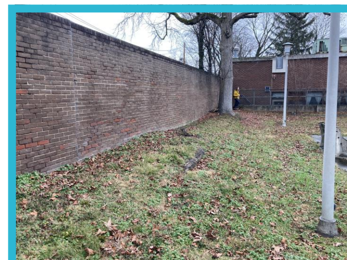
Courtyard Wall – to be removed between existing expansion joints
