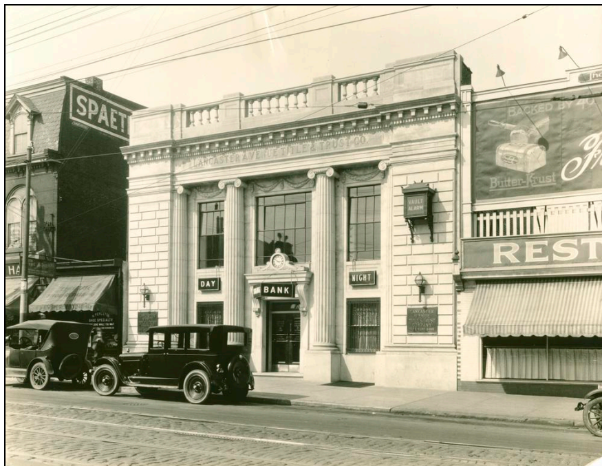
Figure 12: The Lancaster Avenue Title & Trust Company at 3961 Lancaster Avenue in Philadelphia, designed by Charles C. Schweiker and Charles H. Furster in 1923 (from Building a Nation: Indiana Limestone Photograph Collection at Indiana University Bloomington).
