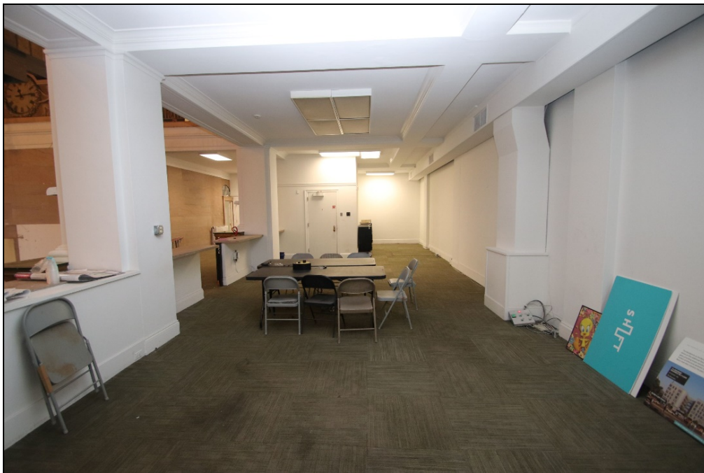
Photo 8: South side of the banking hall, below the mezzanine, looking east.
