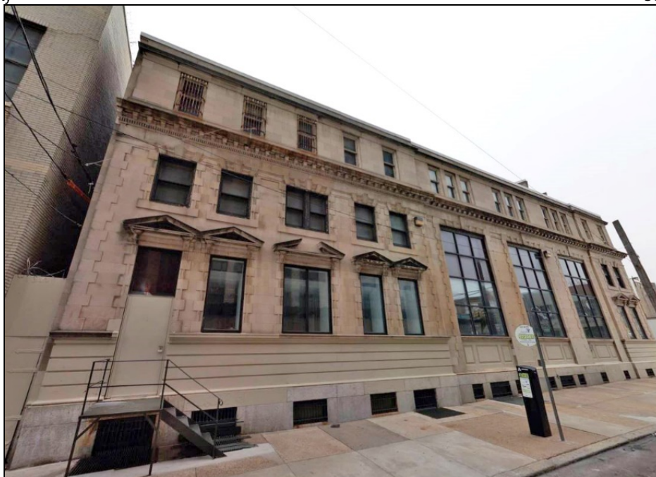
Photo 5: North elevation, facing Airdrie Street, looking southwest.
