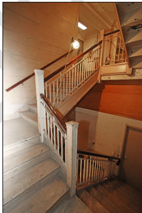
Photo 12: Main stair, looking southwest between the first and second floors.
