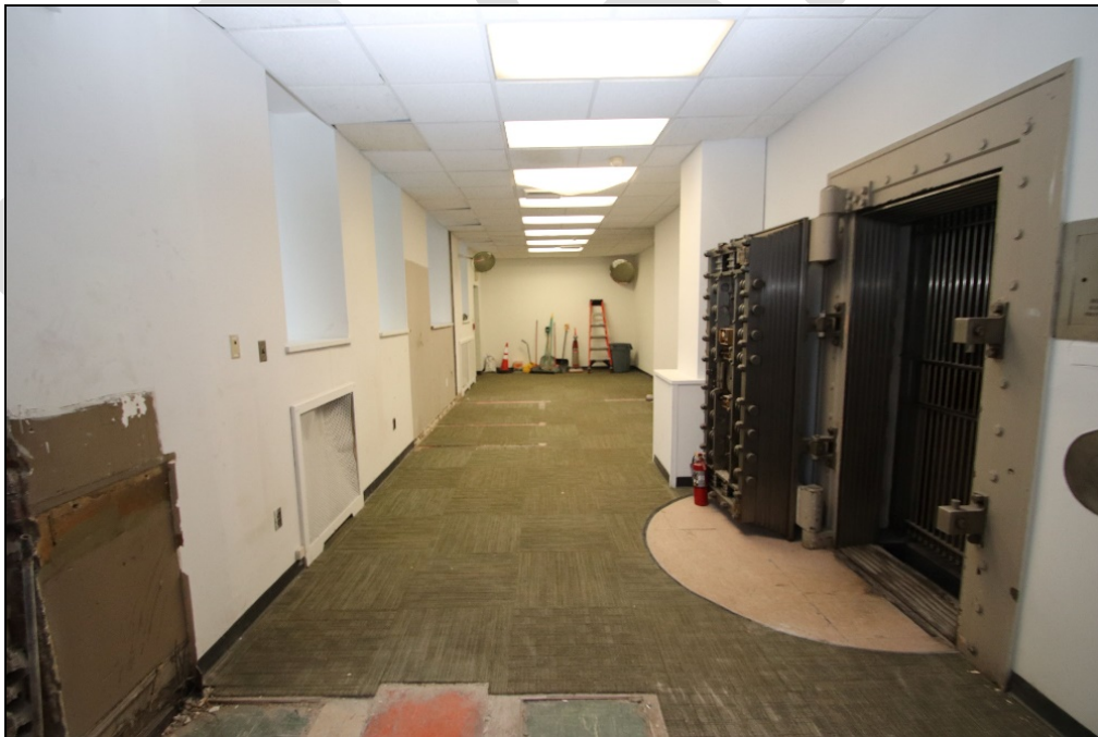
Photo 10: Corridor leading east from the banking hall, south side, looking east.
