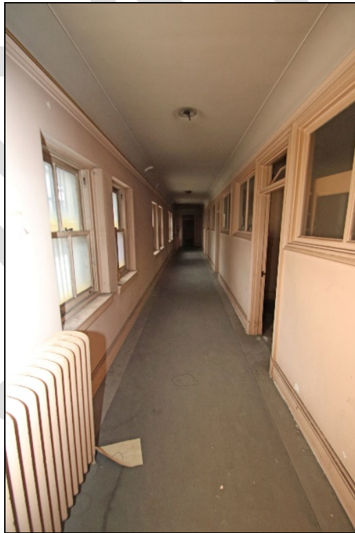
Photo 16 (right): The east-west corridor, looking west.
