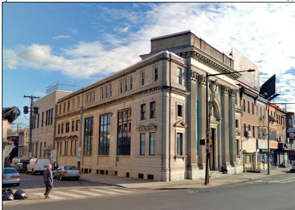
Photo 1: North elevation (Airdrie Street, to the left) and west elevation (Germantown Avenue, to the right), looking southeast from Broad Street.
