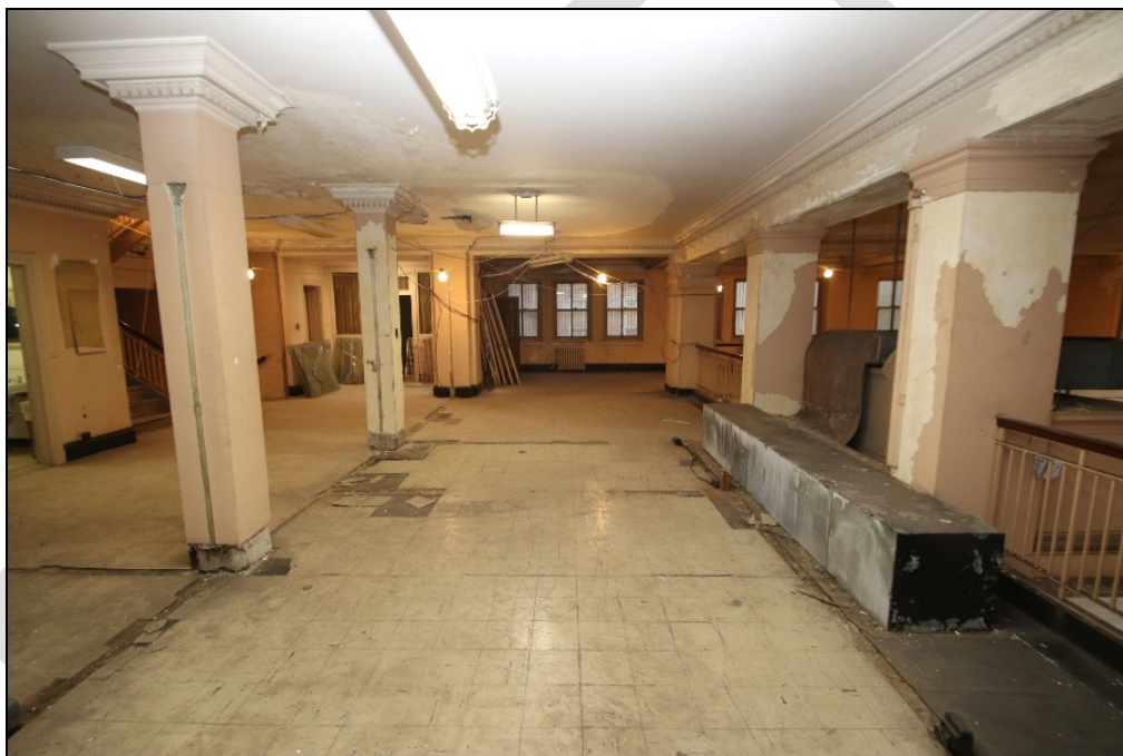
Photo 13: Mezzanine (second floor), east of the banking hall, looking south.
