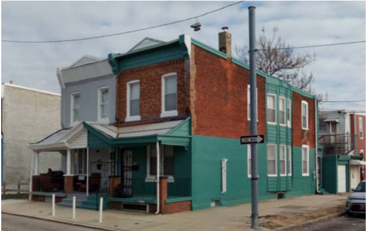
Figure 4. View of the rowhouse at 401 N. Salford Street (on right) looking northeast, December 27, 2022. Source: Cyclomedia.
