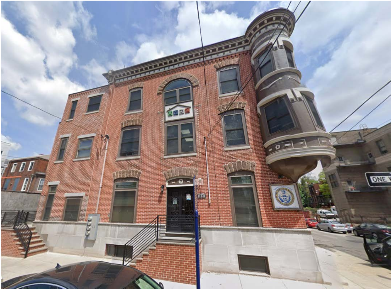
Figure 5: South Elevation of the main black and ell addition. Source: Google Earth
