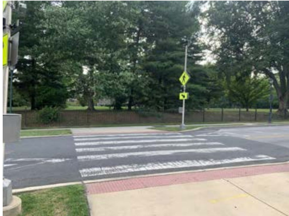
4. Photo at the existing crosswalk across Cardinal Avenue
