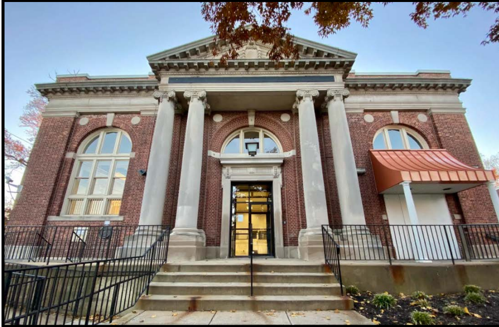
Figure 3. The primary (northeast) elevation of the Pelham Trust Company. Source: Brad Maule, 2020.
