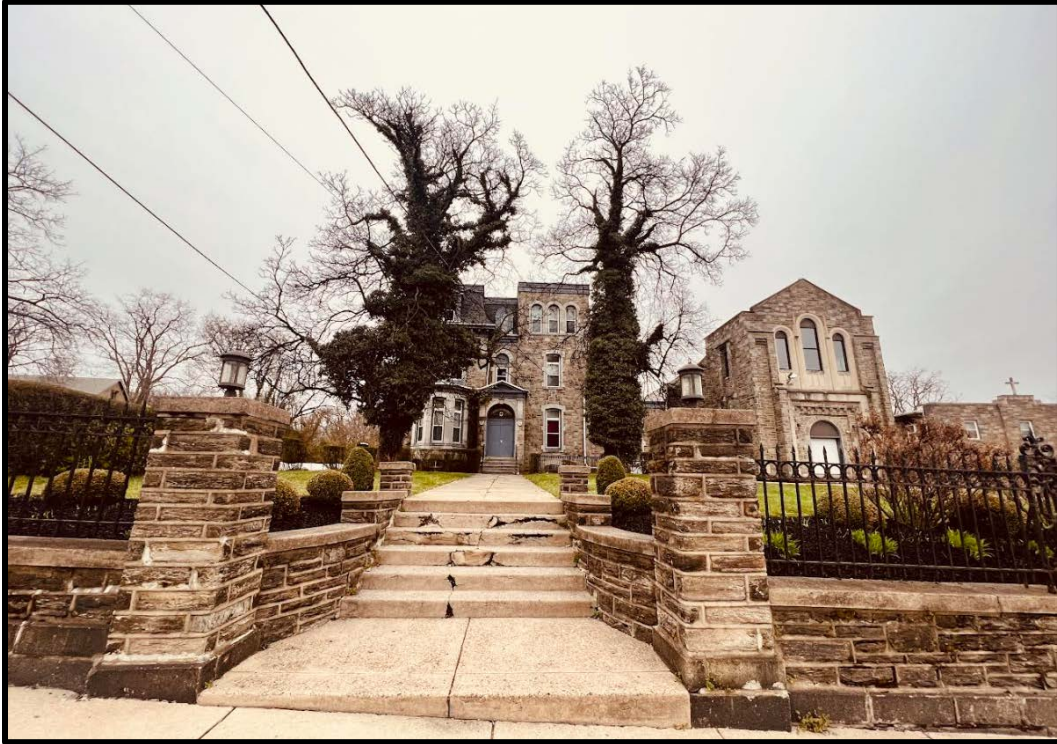
Figure 4. The primary (southwest) elevations of the Adamson Mansion, the Church, the Convent (on far right), and the stone walls and iron fencing along Germantown Avenue. Source: Oscar Beisert, 2022.
