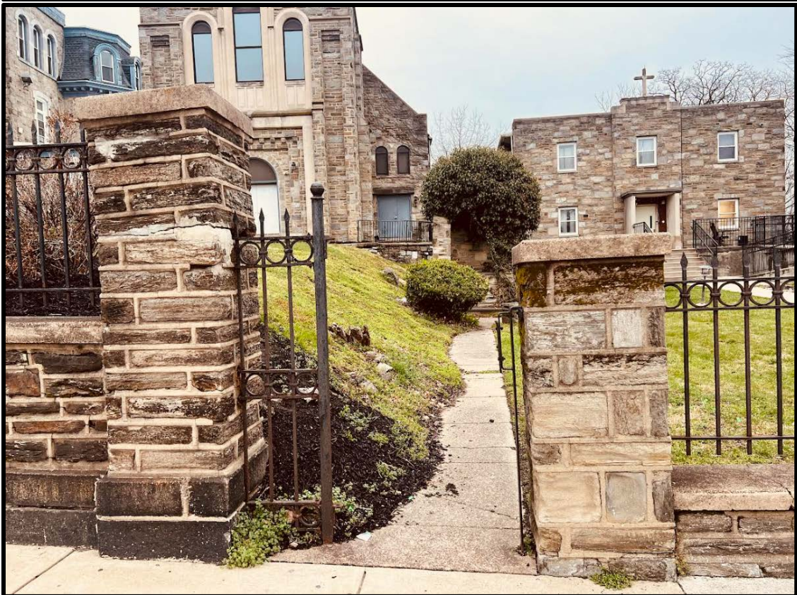
Figure 5. Top: The primary (north) elevation of the Church, the Grotto, and the Rectory through the gateway to the Grotto. Figure 6. Bottom: The side (west) elevation of Building 3. Source: Oscar Beisert, 2023.
