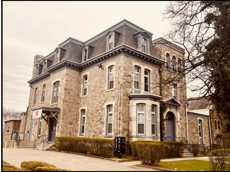
Figure 10. The northwest and primary (southwest) elevations of the Adamson Mansion. Source: Oscar Beisert, 2023.
