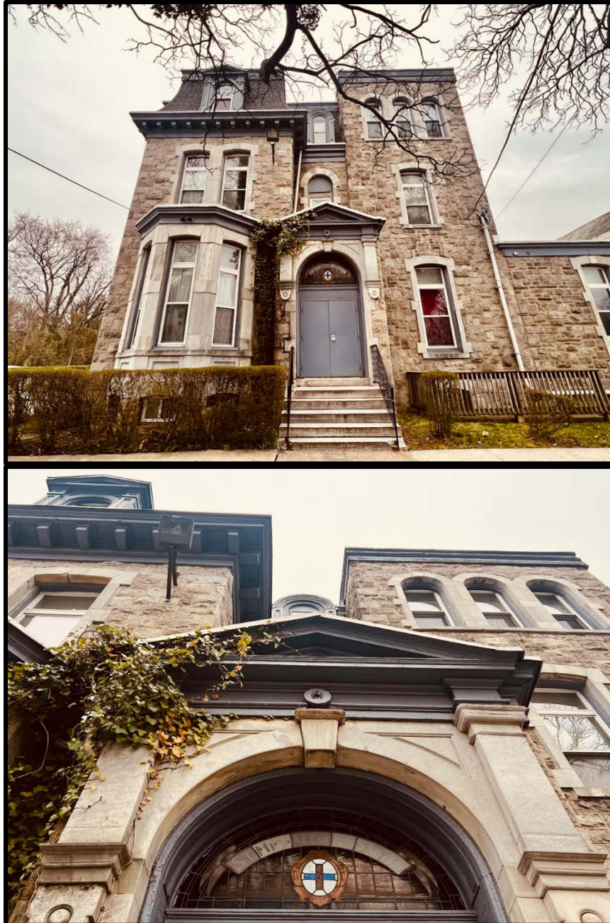
Figure 8. Top: The primary (southwest) elevation of the Adamson Mansion. Figure 9. Bottom: A detail of the primary (southwest) elevation of Adamson Mansion, showing the transom that was installed once the building was renovated to serve the St. Michael of the Saints. Source: Oscar Beisert, 2023.
