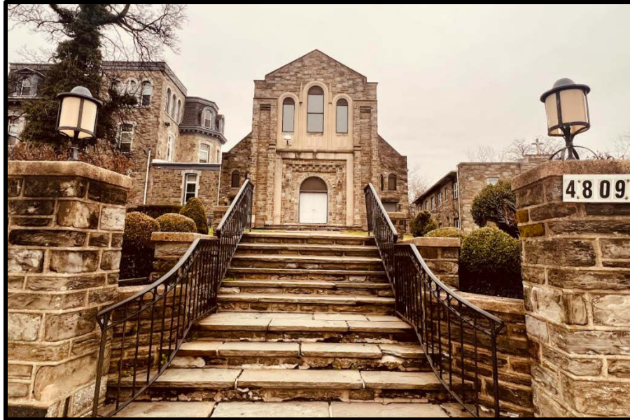
Figure 14. The primary (southwest) elevation of the Church. Source: Oscar Beisert, 2023.
