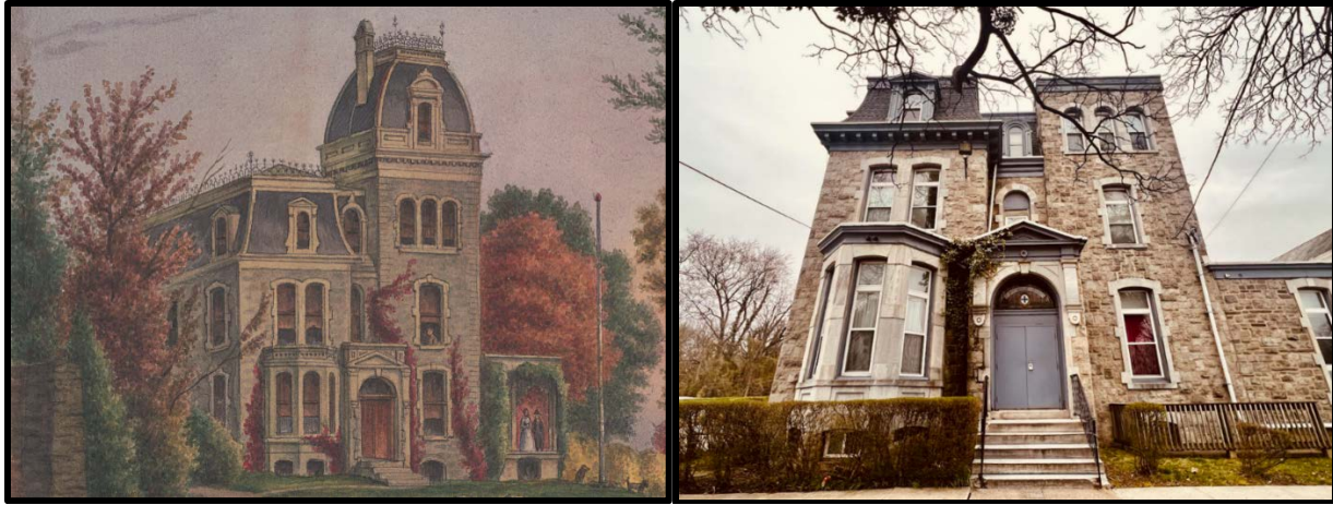
Figure 40. Left: Adamson Mansion, October 1884, by Augustus Kollner. Source: Free Library of Philadelphia. Figure 41. Right: The primary (southwest) elevation of the Adamson Mansion. Source: Oscar Beisert, 2023.
