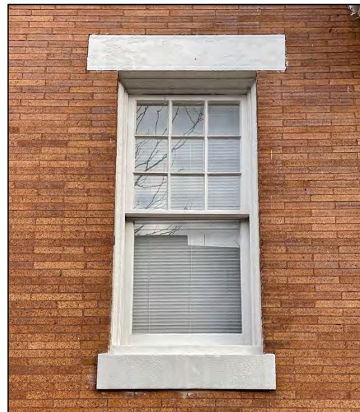
Fig. 12. Typical 9/1 double hung window at the west elevation.
