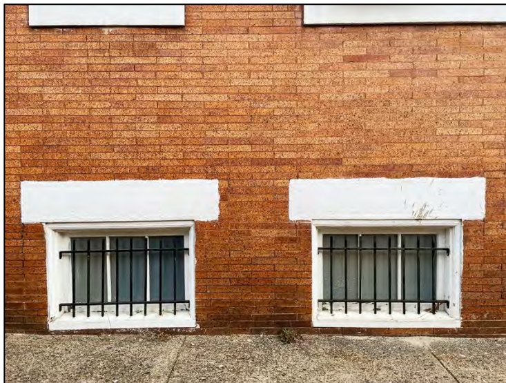
Fig. 9. Typical basement windows at west elevation.
