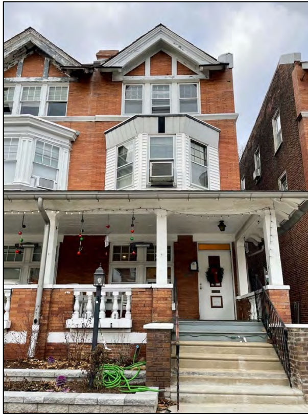
Fig. 4. South & primary elevation of 4949 Walnut Street.
