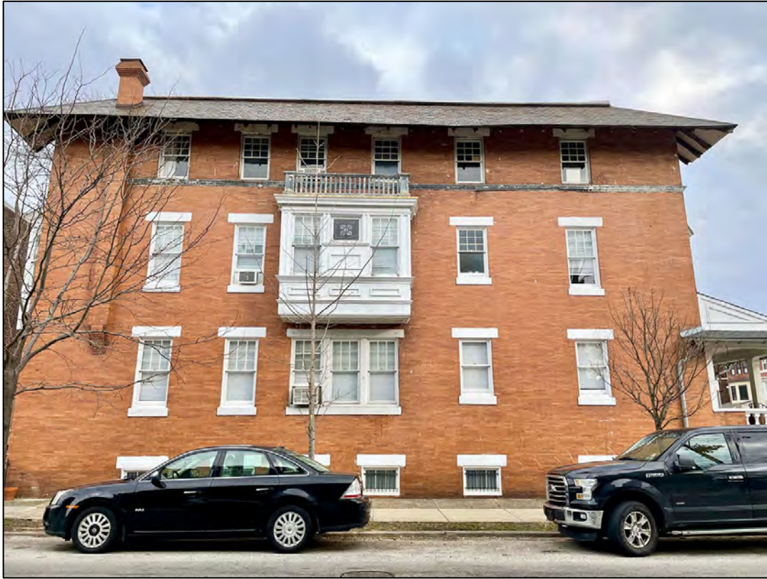
Fig. 10. West elevation of 4951 along S. 50 th Street.
