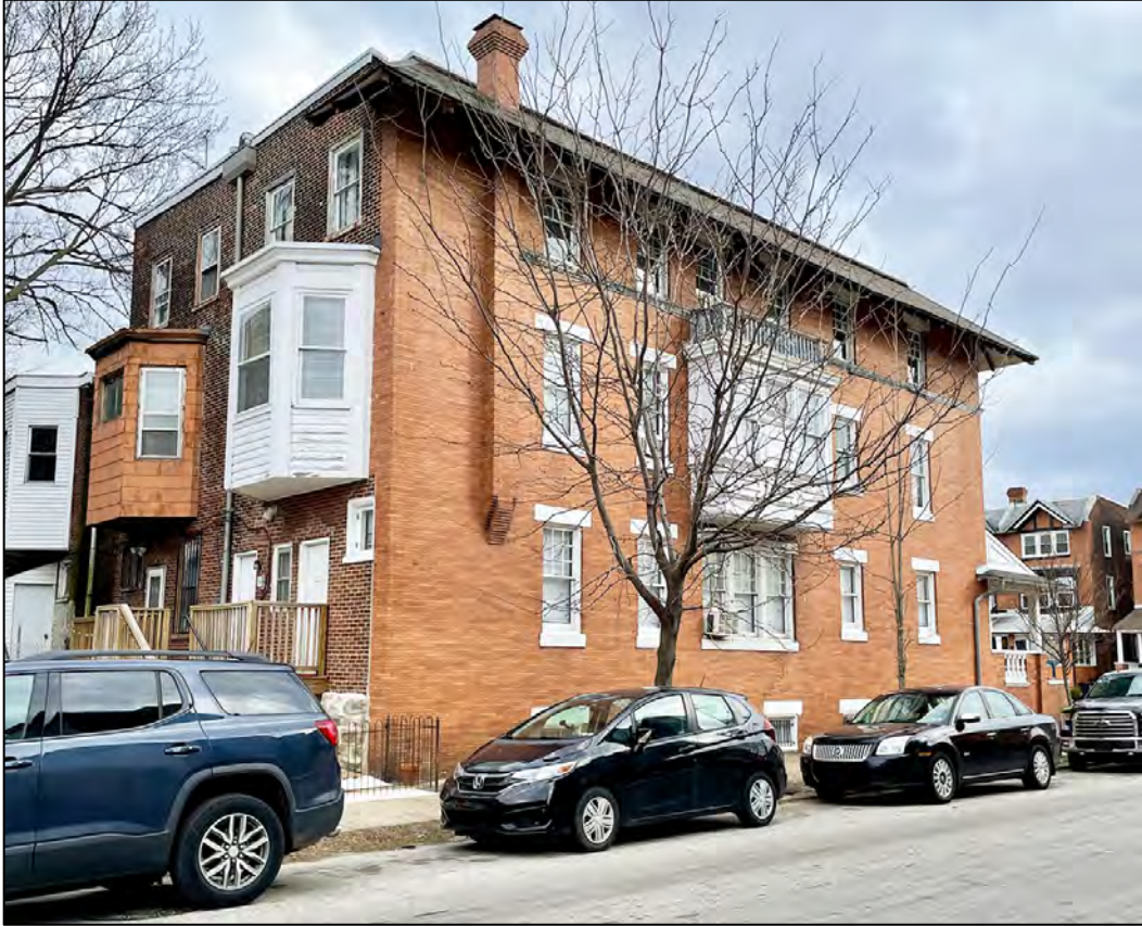
Fig. 13. Northwest corner of building showing rear of both properties and west elevation.
