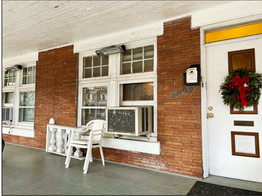
Fig. 5. South façade at shared porch showing the entry door to 4949.
