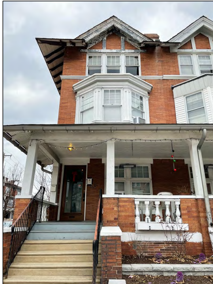
Fig. 6. South (primary) elevation of 4951 Walnut Street.
