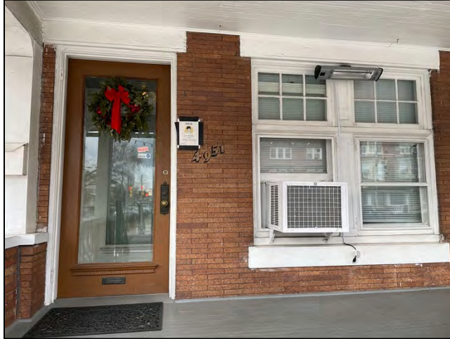
Fig. 7. South façade at entry porch.
