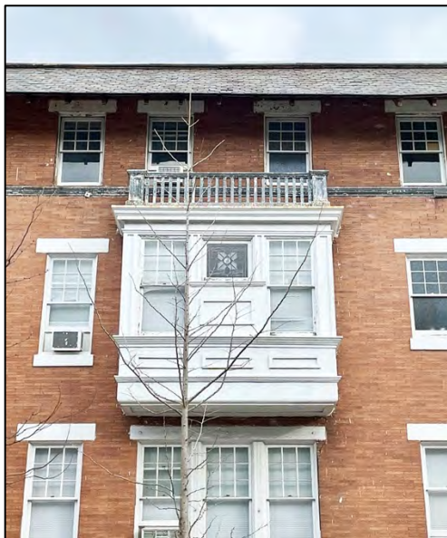
Fig. 11. Close up of second story window bay at west elevation.
