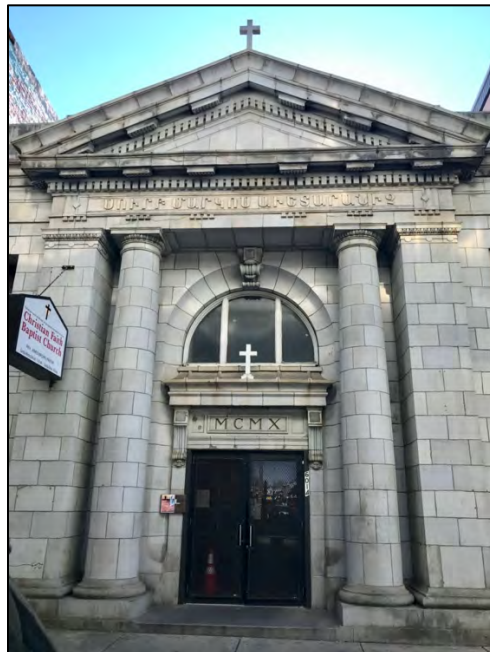
Fig. 18. North elevation of the former Haddington Title and Trust building on Market Street. Later an Armenian church (see script in entablature), now a Baptist church. Photo by A. Lambert, 2/11/2023.
