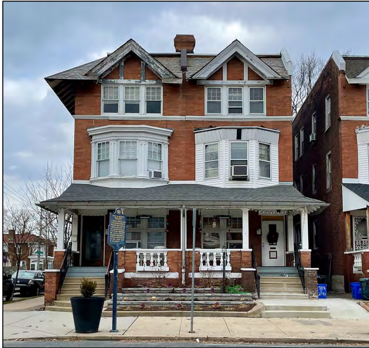
Fig. 3. South elevation of 4949 & 4951 Walnut Street.
