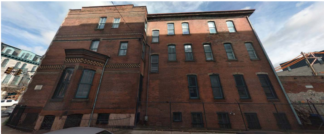
Figure 4: Fitzwater Street Elevation. Image from Cyclomedia.phila.gov .
