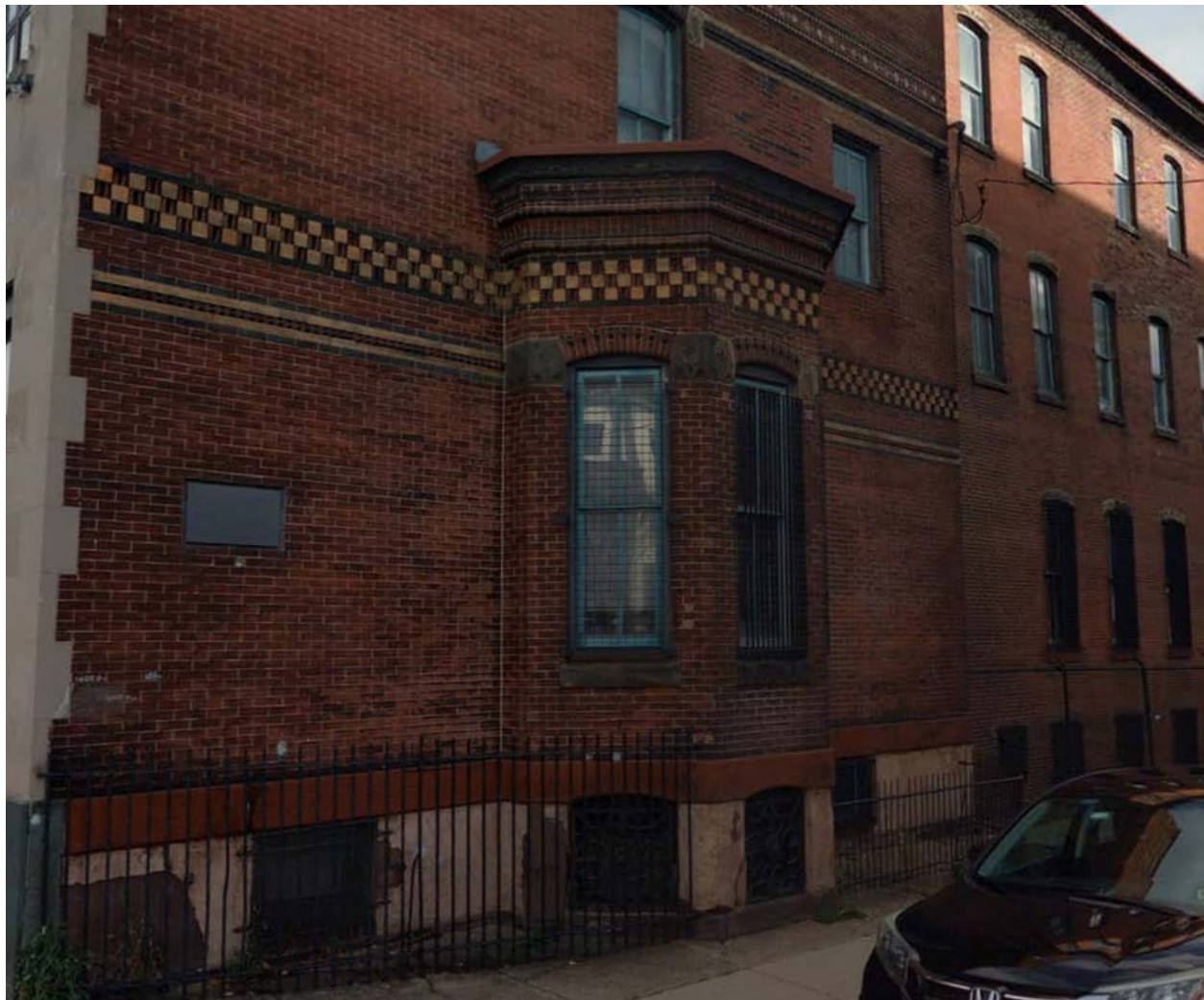
Figure 5: The Fitzwater Street Bay. Image from Cyclomedia.phila.gov
