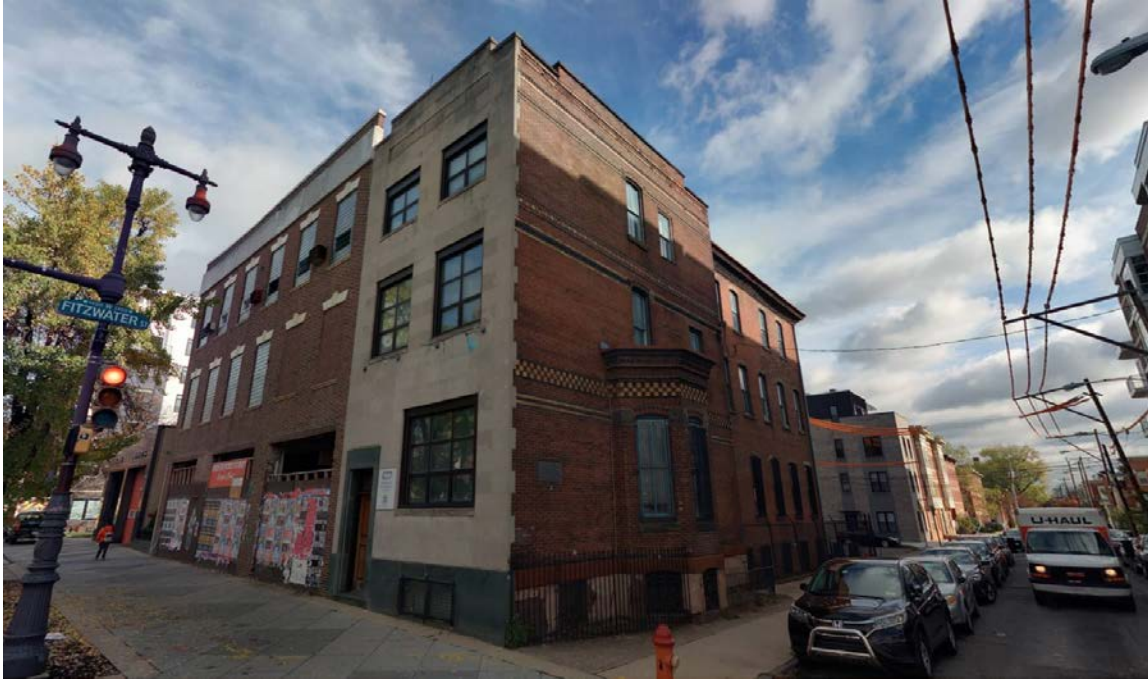
Figure 1: View of 731 S. Broad Street, looking Northeast. Image from Cyclomedia.phila.gov
