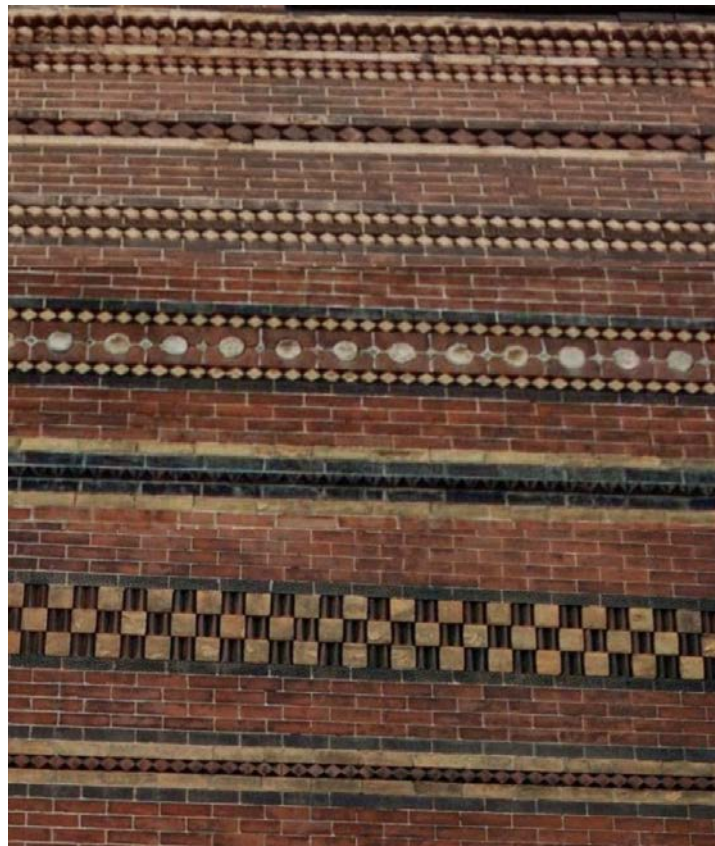
Figure 18: Composite image showing the decorative brick courses. Images from Cyclomedia.phila.gov , composition by Ted Maust.
