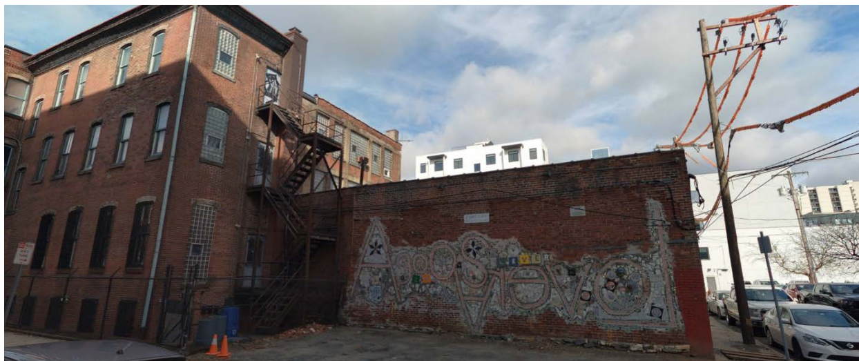
Figure 14: The rear and parking lot of 731 S. Broad Street. Image from Cyclomedia.phila.gov
