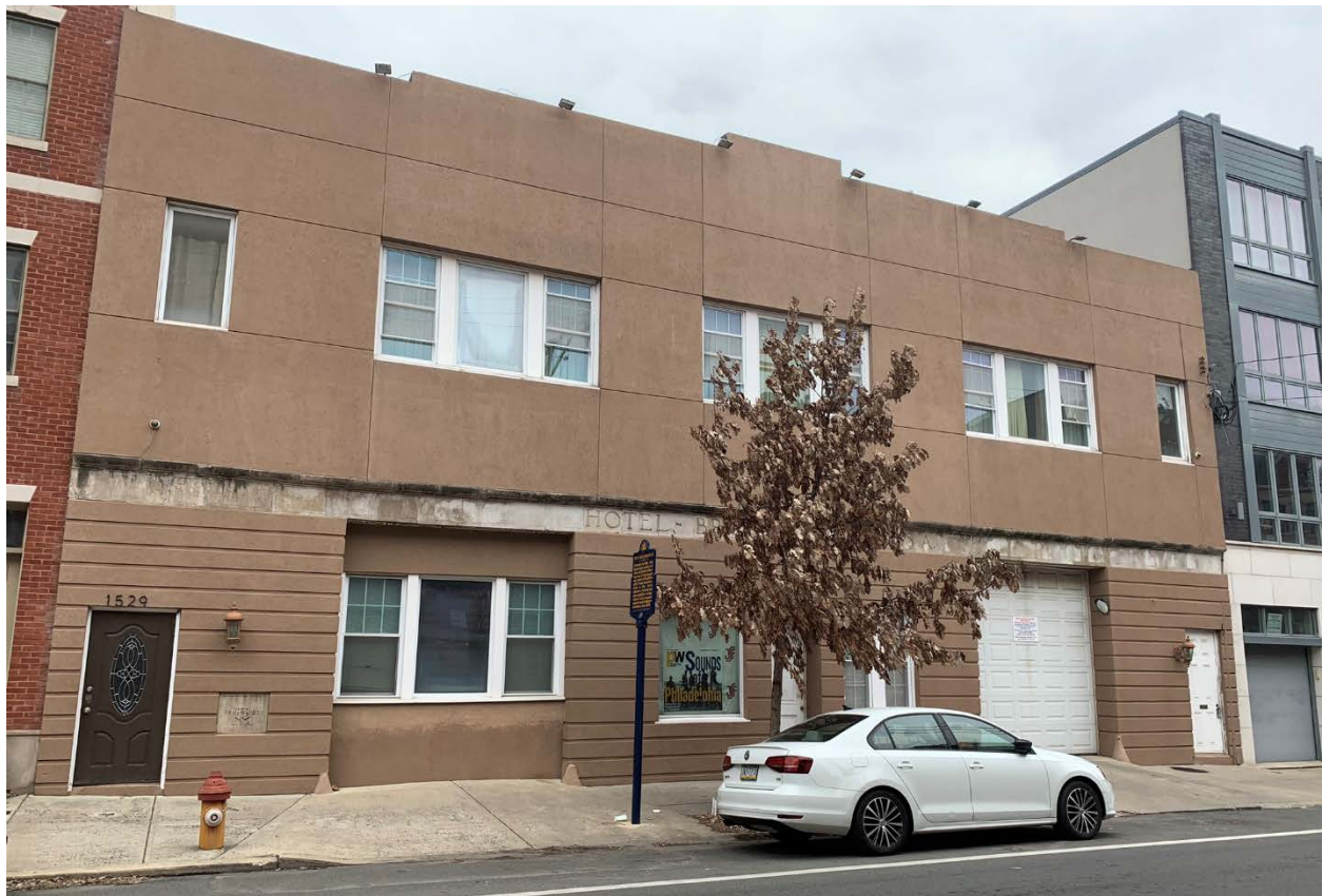
Figure 1. 1523-29 Bainbridge Street front façade. February 2023.
