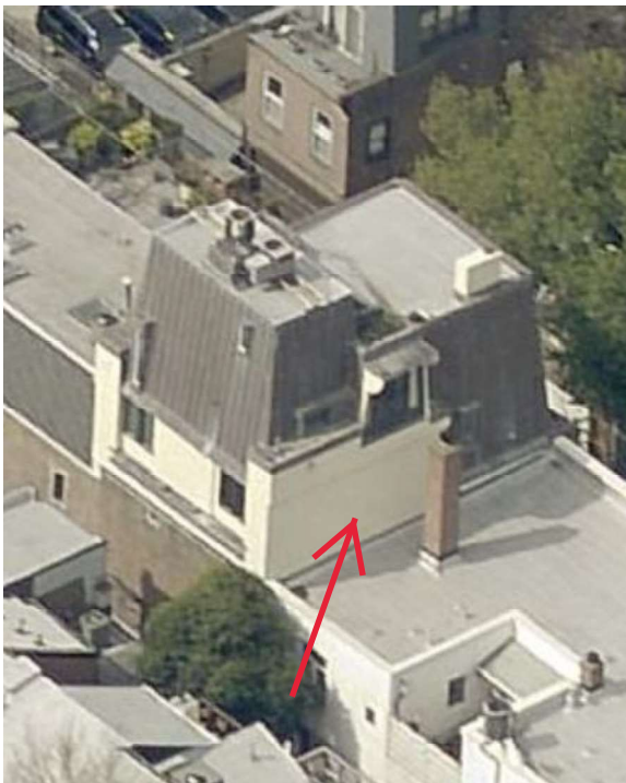
Figure 13: The north elevation has a projecting balcony matching the one on the south elevation of mansard.
