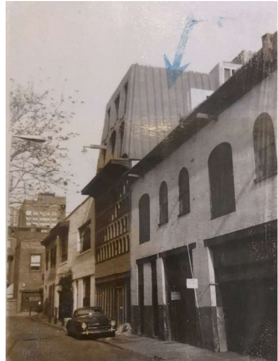
Figures 34: 1971 Photograph. The first level in front is still boarded up and appears unfinished.
