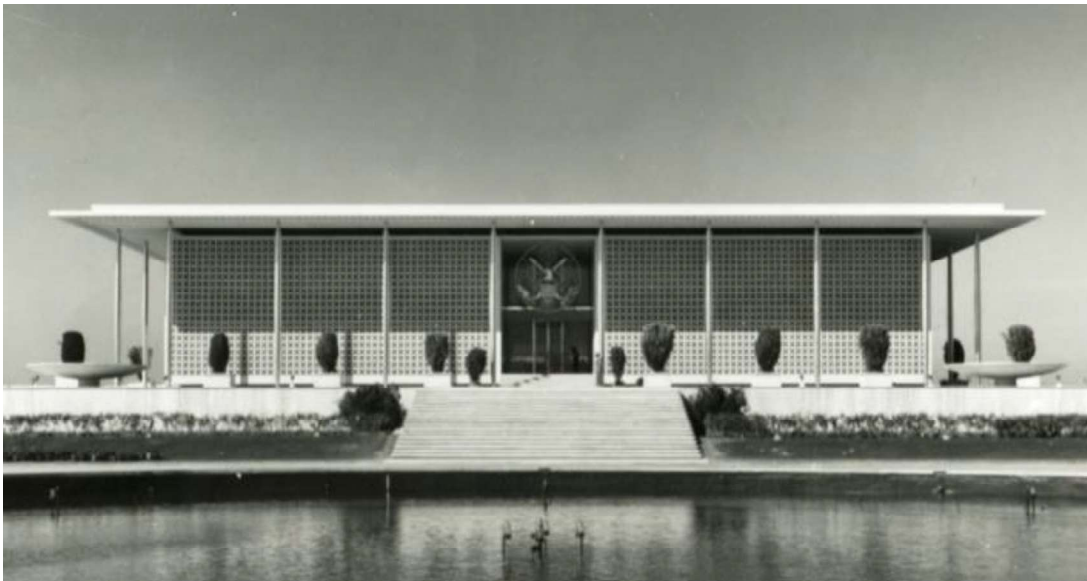
Figure 45: U.S. Embassy New Delhi, India. Completed 1959. Architect Edward Durrell Stone. Photo credit: Docomomo US, https://www.docomomo-us.org/register/u-s-embassy-in-new-delhi .
