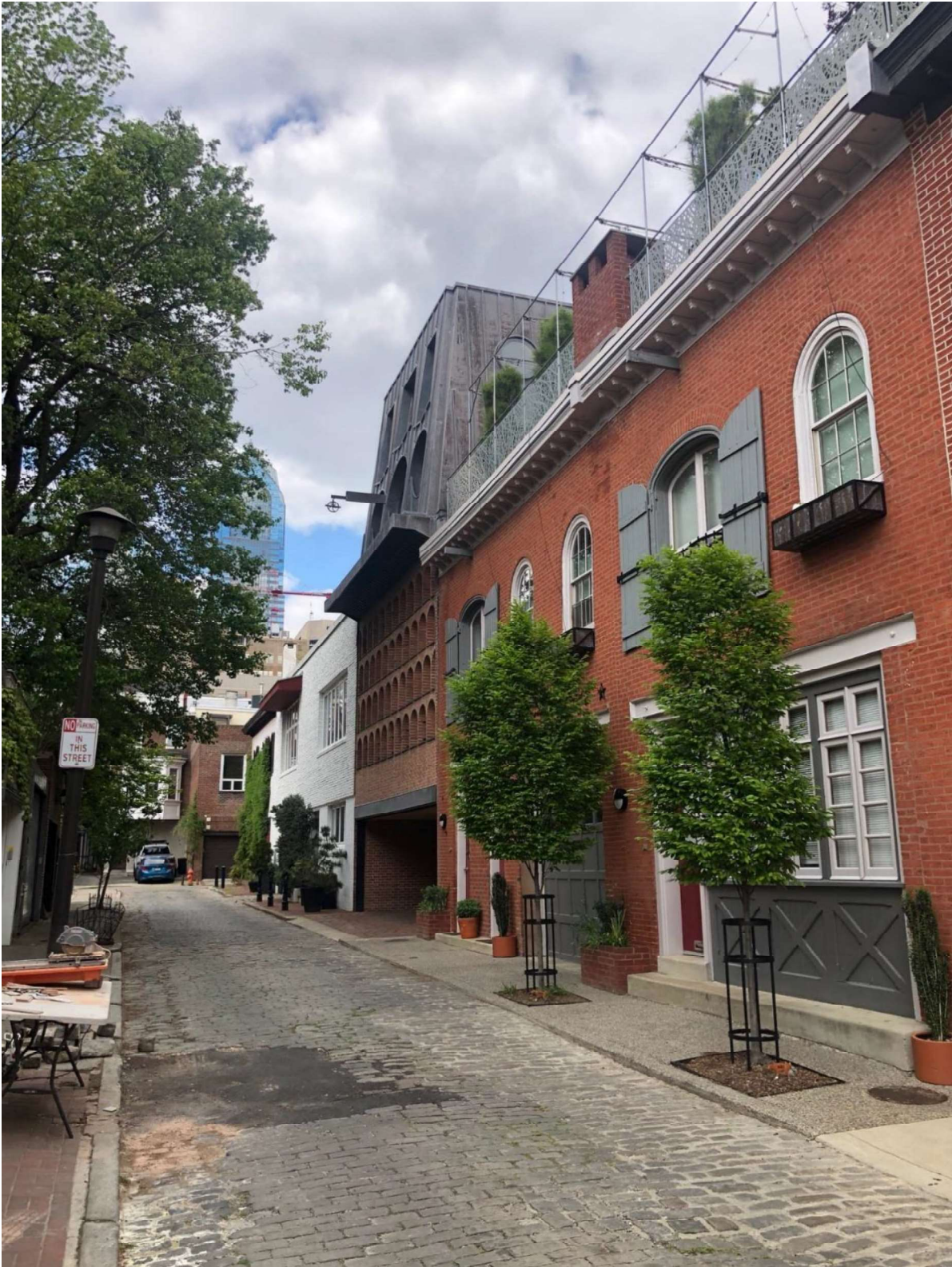
Figure 5: View looking north up S. Chadwick Street toward the intersection with Cypress Street. The east side of the street was developed in the nineteenth century primarily with two-story stables. The original stable at 307 S. Chadwick Street was never fully demolished. Party walls and floors (and joists) appear to have been incorporated into the altered building.
