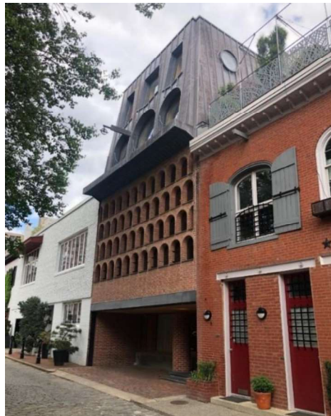
Figure 1: View looking north along S. Chadwick Street. The brick section of the façade stops below the cornice and is at the height of neighboring brick buildings. The majority of buildings on the west side of S. Chadwick Street are former stable buildings constructed in the late nineteenth century. Figures 1-10 were photographed on April 26, 2023, by Historical Commission staff.
