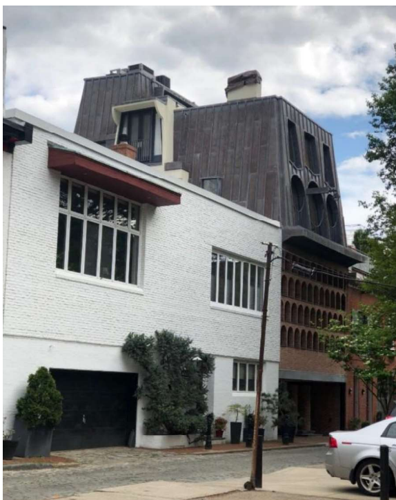
Figure 2: View looking south down S. Chadwick Street. The mansard rises prominently above the neighboring buildings. The chimney, Juliet balcony, and roof mezzanine on the building's north wall are visible from street level.
