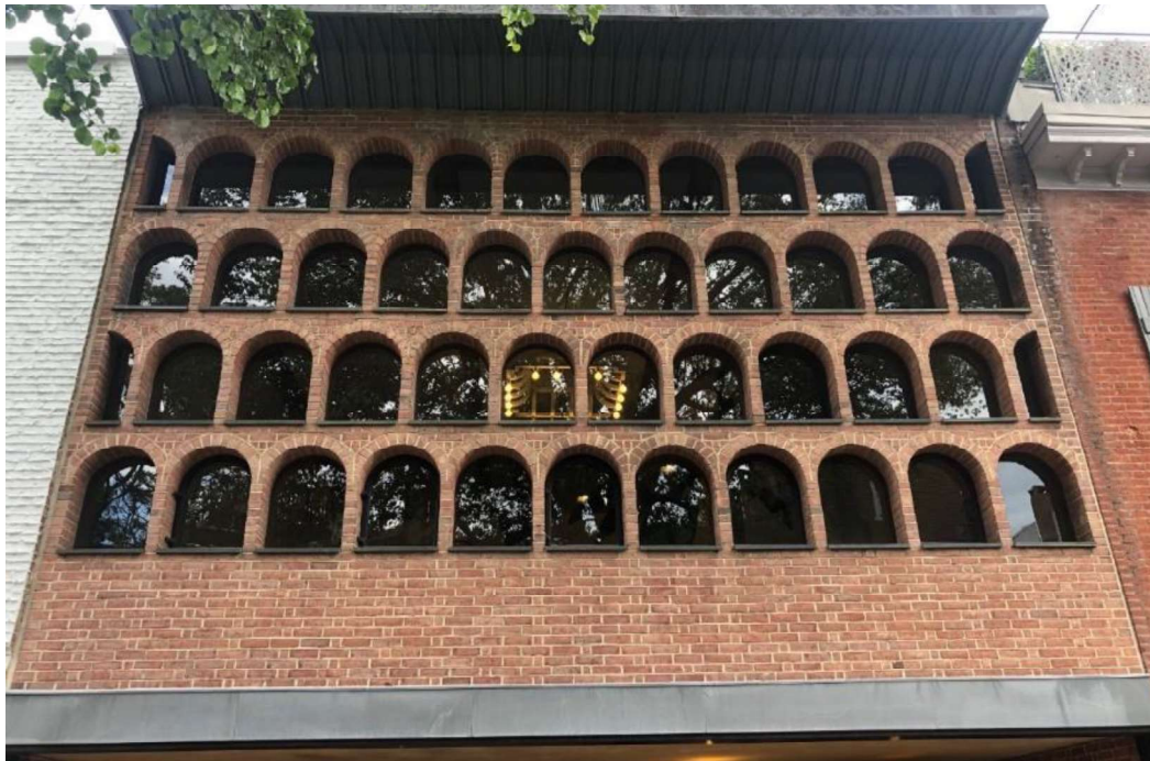
Figure 10: Brick laid in Flemish Garden Wall bond is visible above the first floor. Four rows of tiered rounded arches rise up toward the cornice. A patterned, cantilevered cornice tops the brick arches. Patterned lines accentuate the appearance of the cornice pushing (and slightly curving) away from the façade.
