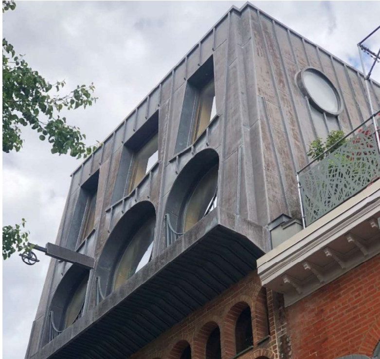
Figure 9: The front of the mansard features oversized circular and pentagonal window openings. A pulley system is installed and projects outward. While the pulley may have been a practical tool for moving large items to the upper levels, it is also a nod to the past.
