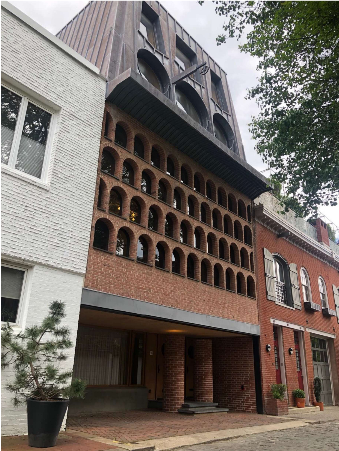
Figure 4: A full view of the front façade. Weise's skill with Modernist residential design is seen on the first floor. He sets the wall and entrance back to create a shadowed area at the building's base. This encourages a visual illusion of the upper levels floating above.
