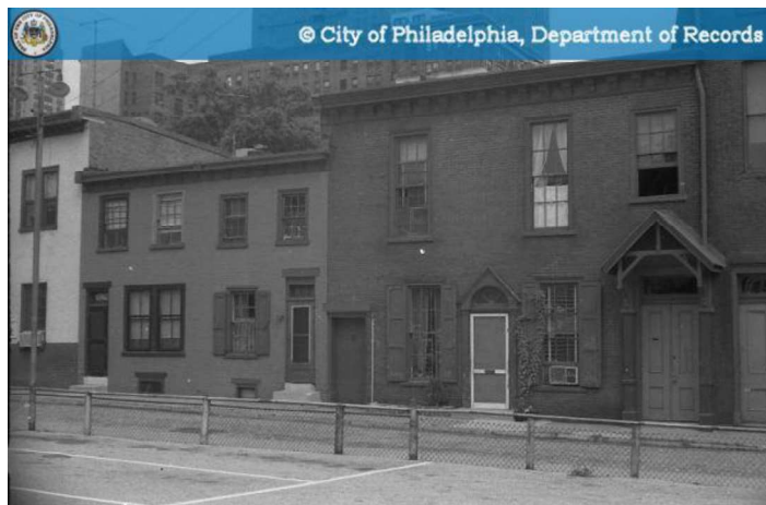
Figure 18: No photographs of the stable at 307 S. Chadwick Street have been located. 317, 319, and 321 S. Chadwick Street are shown in undated photo, circa 1960s.
