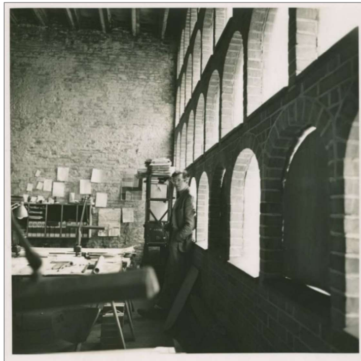
Figure 15: Frank Weise at 307 S. Chadwick Street. He used the second floor as his studio. The former stable's party wall and rafters are visible in this photograph taken circa late 1960s. Undated photograph, Frank Weise Collection, Architectural Archives of the University of Pennsylvania.
