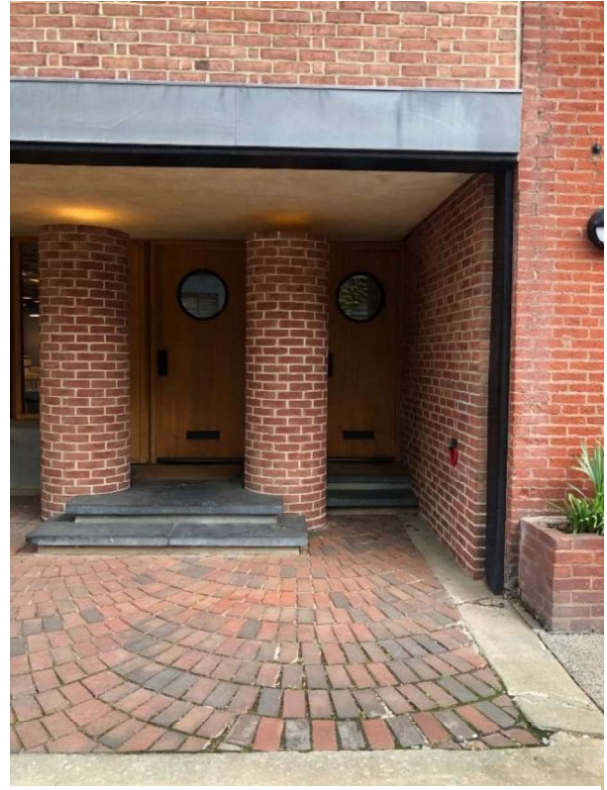
Figure 7: The two entrances are accessed by blue stone steps. The entry doors are wood with circular windows. Separate entryways for the studio and living areas allowed for privacy between the spaces.
