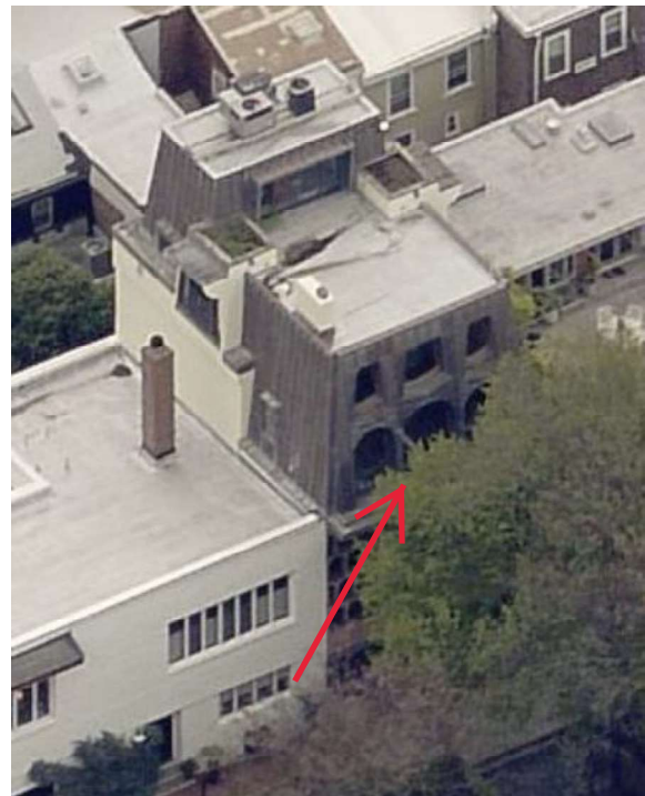
Figure 14: A view showing the top of the front facade and roof mezzanine. The top of the mansard has a flat roof.
