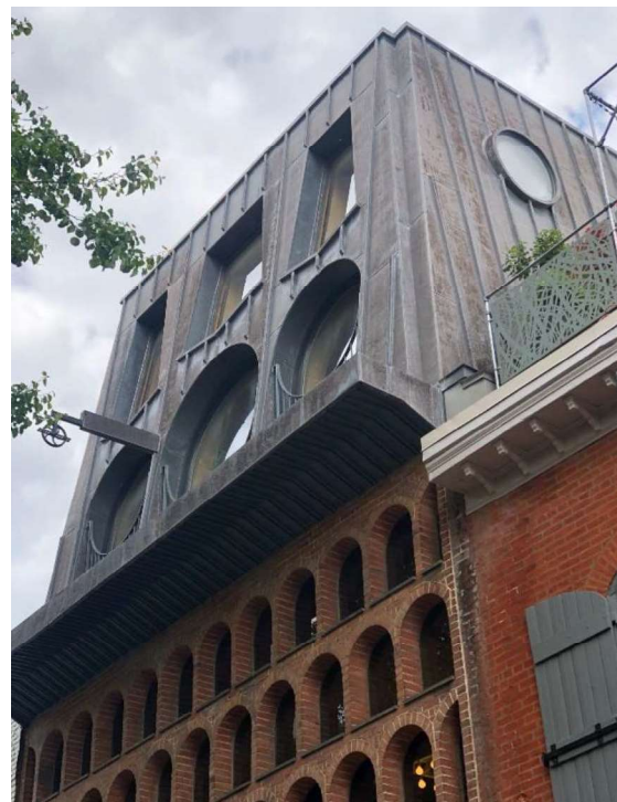
Figure 3: The mansard's front façade features oversized window openings made up of a one row of circles and an upper row of pentagons. A port hole type window on the south façade was a later alteration by the architect.
