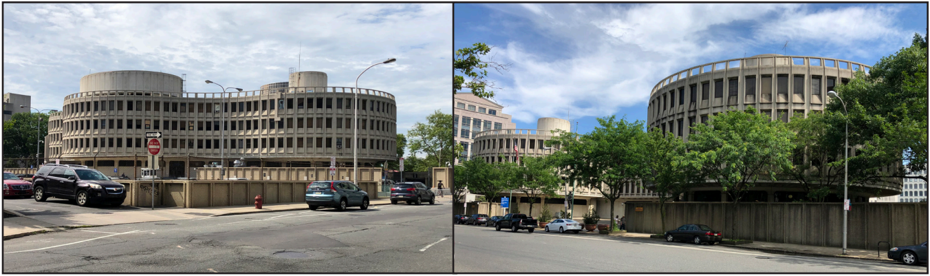
Plate 1 (left): View of the south elevation of the Philadelphia Police Headquarters, from Seventh Street (Source: Allee Davis, June 2019)
