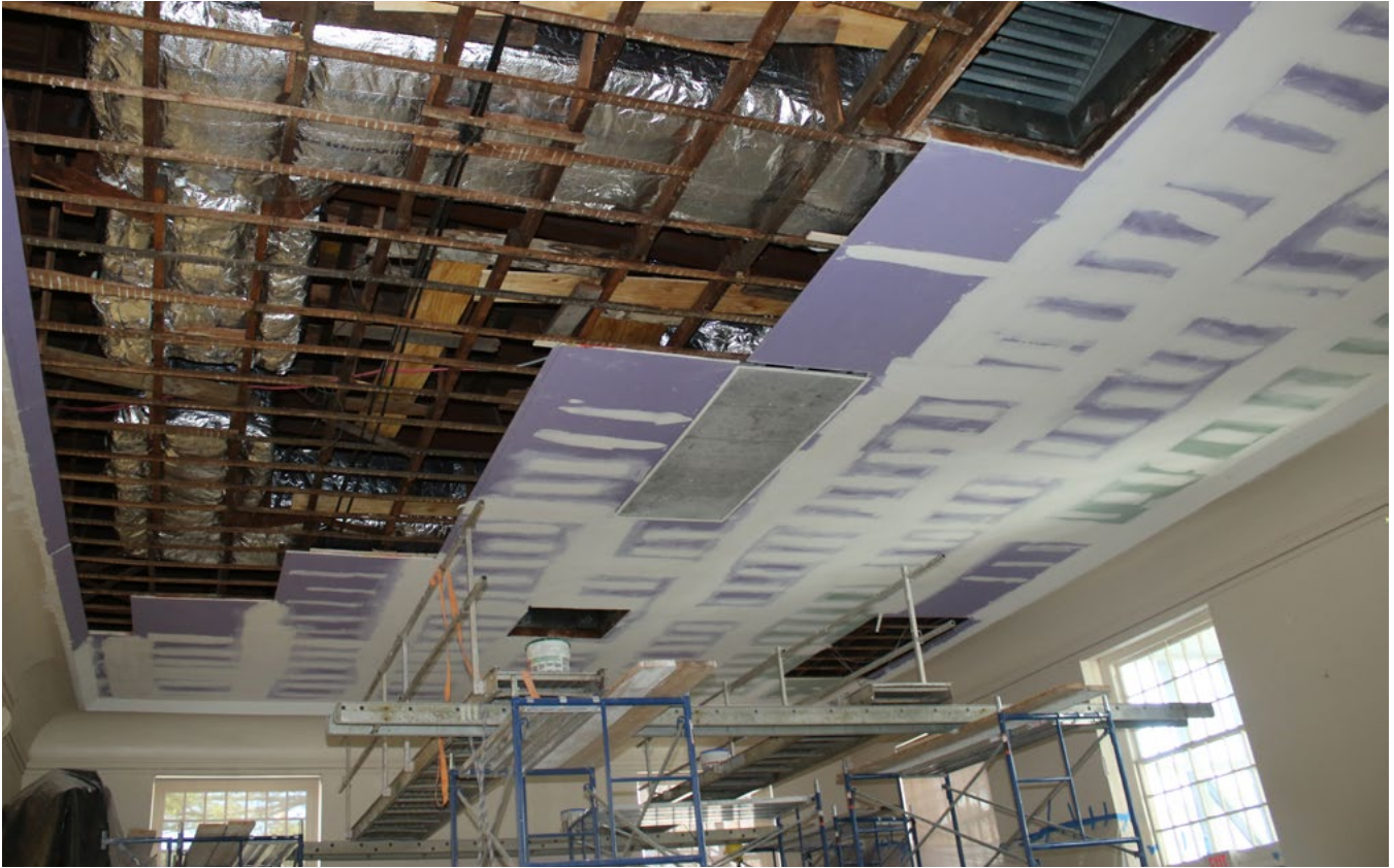
NEW CEILING AT THE CARNEGIE LIBRARY CHESTNUT HILL
