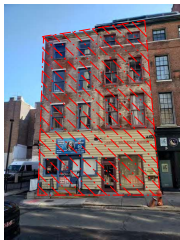
2ND STREET FRONT VIEW, EXISTING
