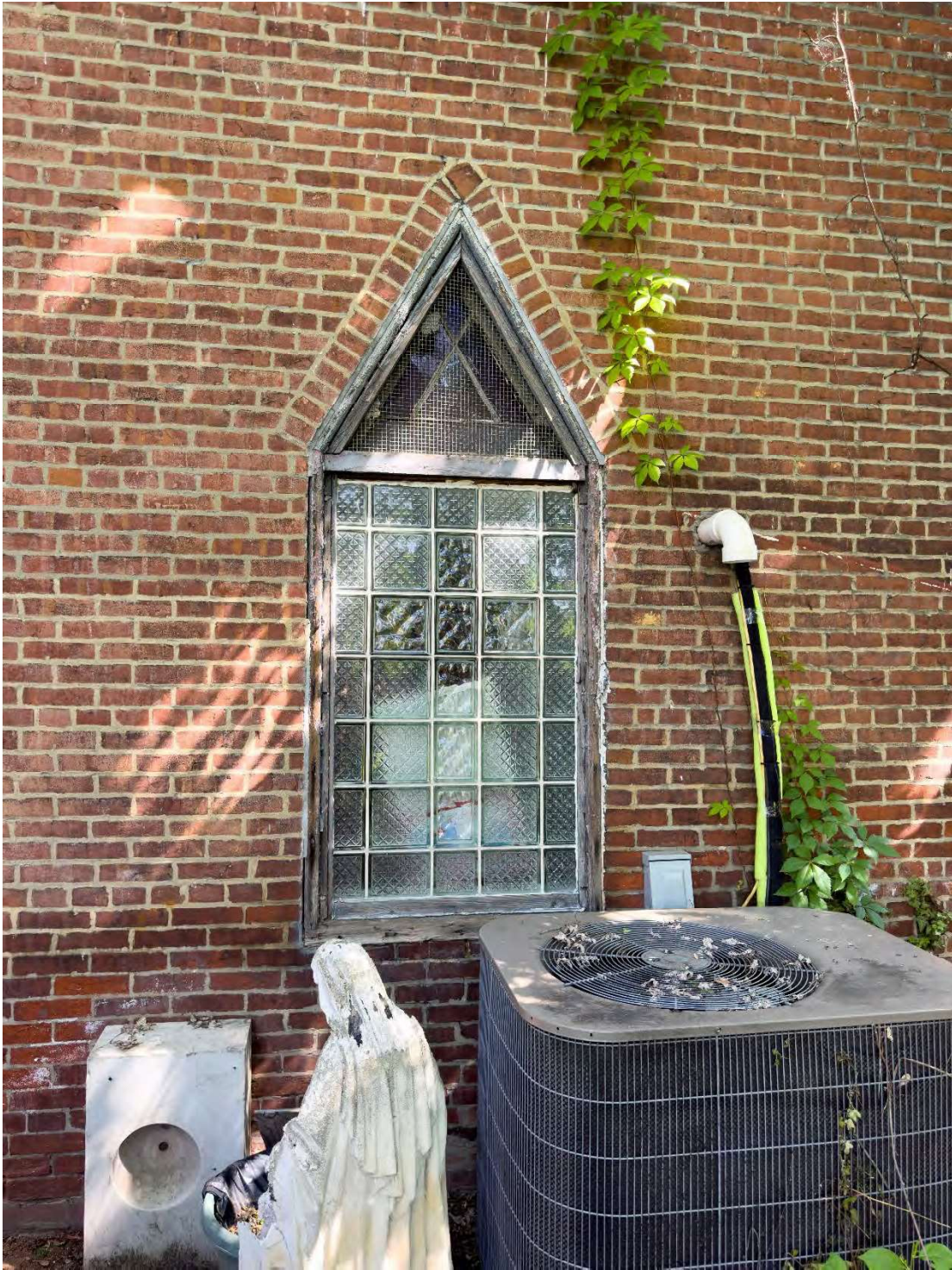
Figure 8. Detail of easternmost window opening. Notice the leaded stained glass in the triangular opening.
