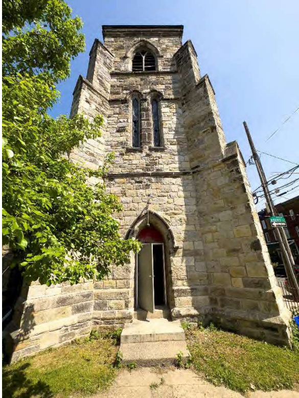
Figure 5. View of belltower looking North
