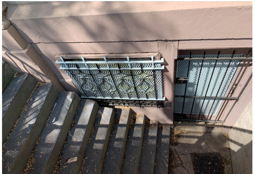
Detail of basement access, photo by author
