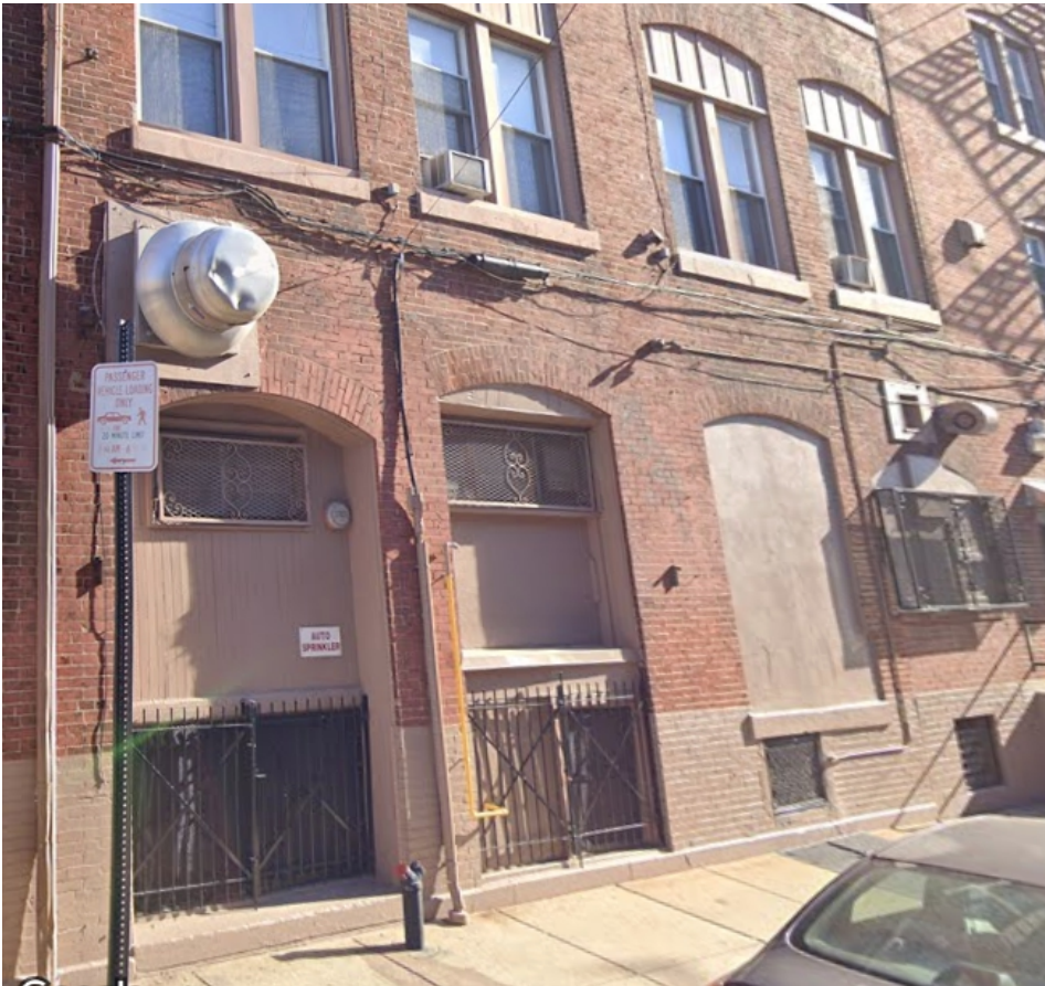
Ground story of 764, Google
