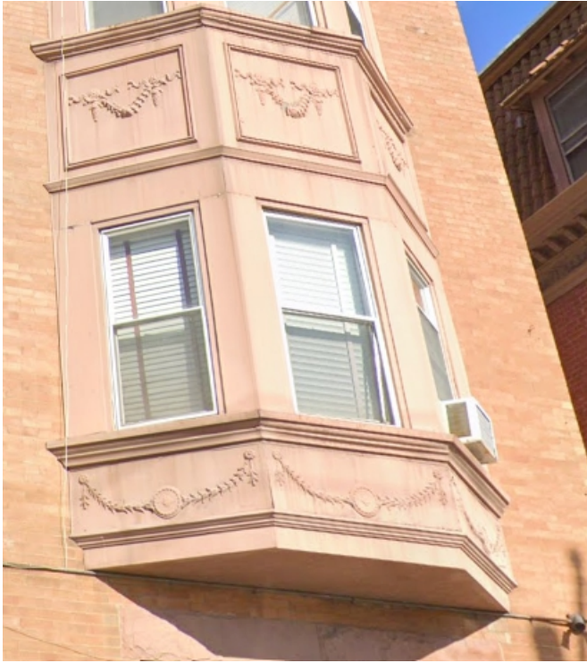
Detail of oriel and cornice bracket, Google
