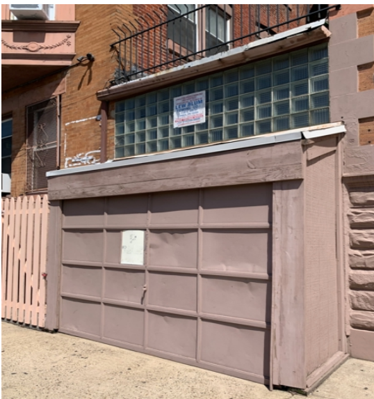
Detail of garage, photo by author
