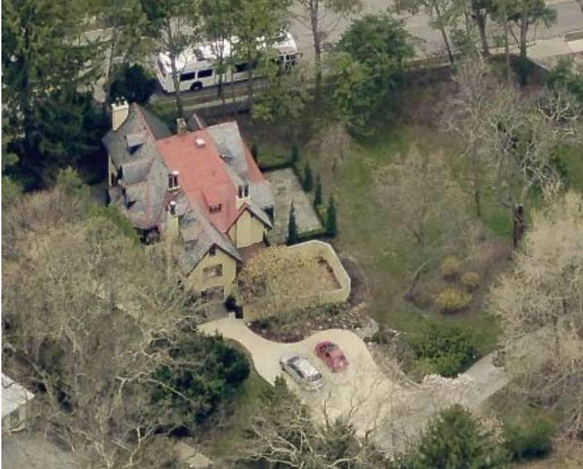
Figure 11: Aerial photo of 150 Bethlehem Pike with Bethlehem Pike at the top, showing the East elevation. Image from Pictometry.phila.gov.
