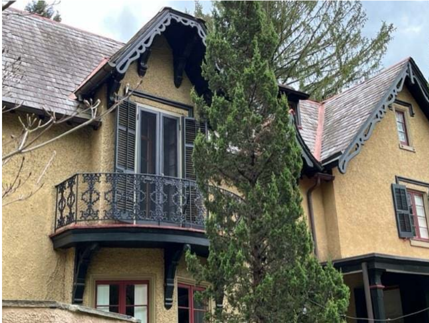
Figure 13: Detail of the North elevation, showing the corbeled Juliet balcony below the clipped gable. Photo by Massimo Cristofanilli.
