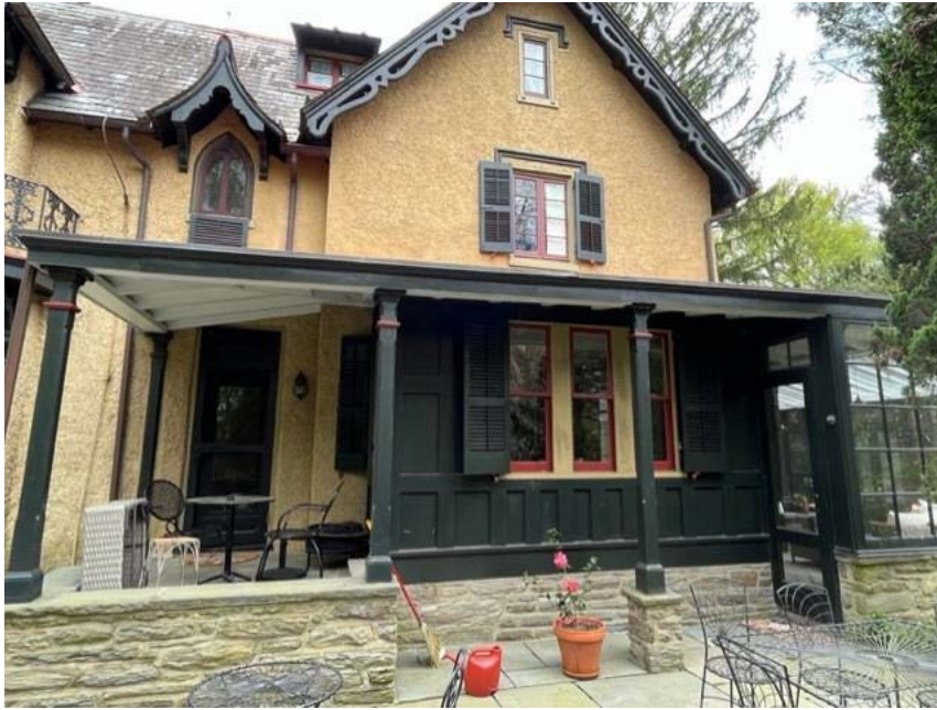
Figure 14: Detail of the North elevation, showing the sloped gable dormer, shed dormer, porch, and exterior wood paneling. Photo by Massimo Cristofanilli.
