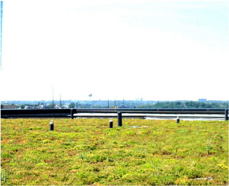
Extensive Green Roof System
