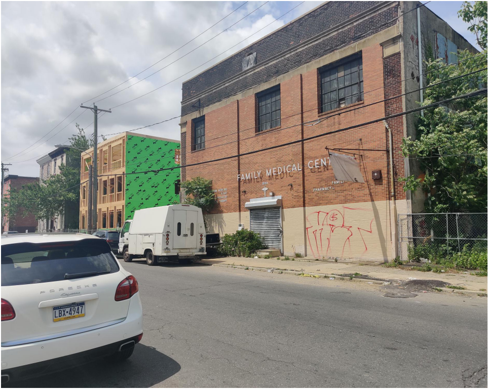
2 - Looking West on N 22nd St
