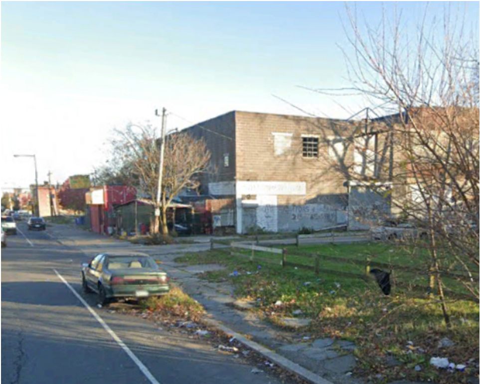
6 - Looking South East on the corner of W Diamond St
