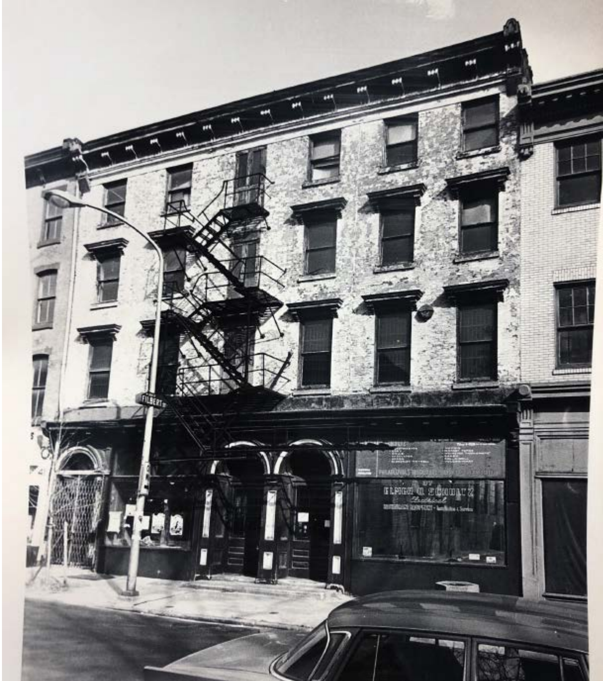
Figure 5: 1977 designation photograph of 37-39 N. 2 nd Street. Historical Commission files.
