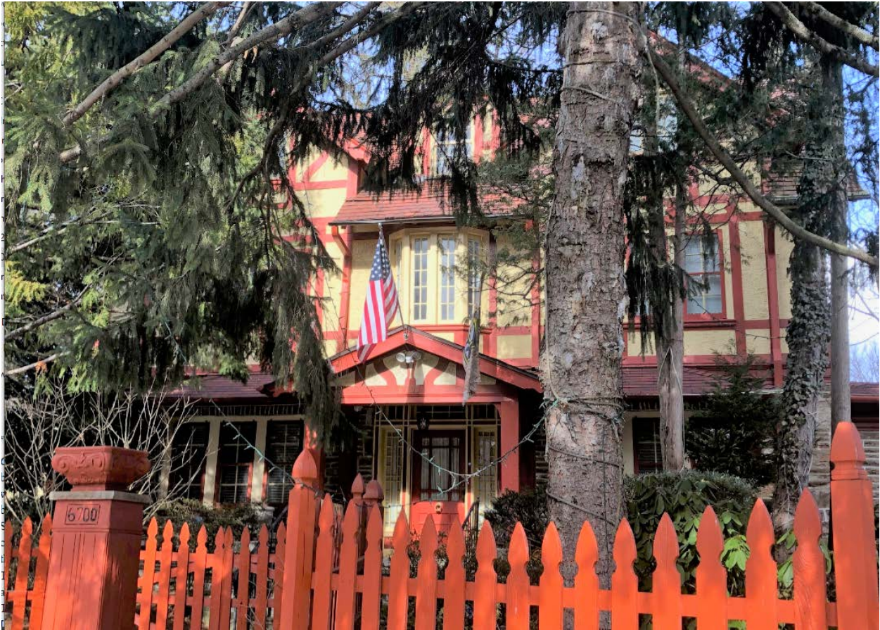
Figure 6: Front façade of 6700 Lincoln Drive, from McCallum Street, February 2023.
