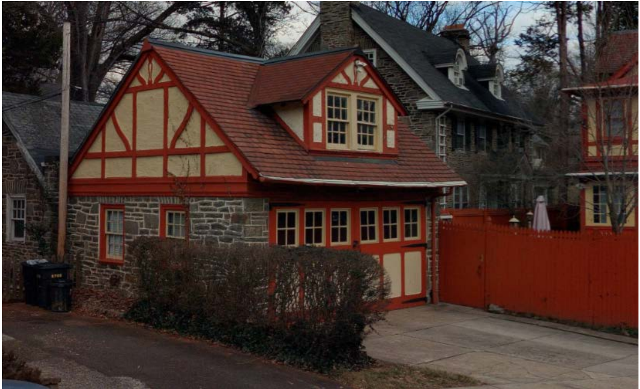
Figure 12: South and west elevations of the garage. Source: Cyclomedia, January 2023.
