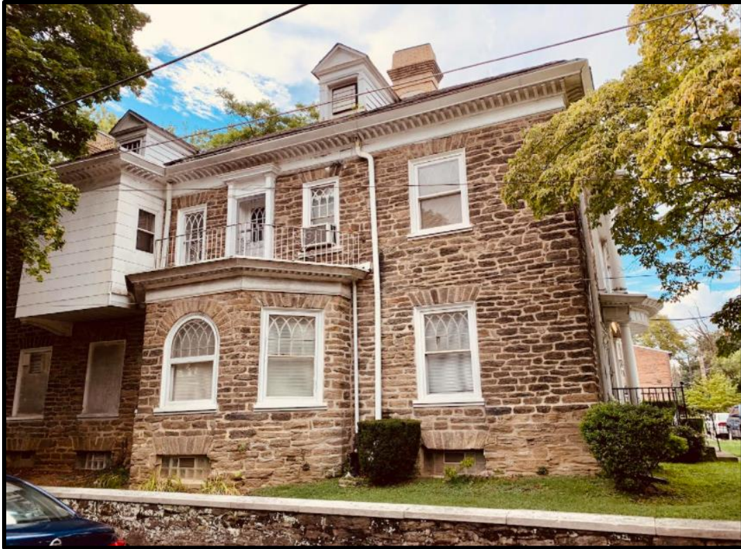
Figure 9. The southeast elevation. Source: Oscar Beisert, 2021.
