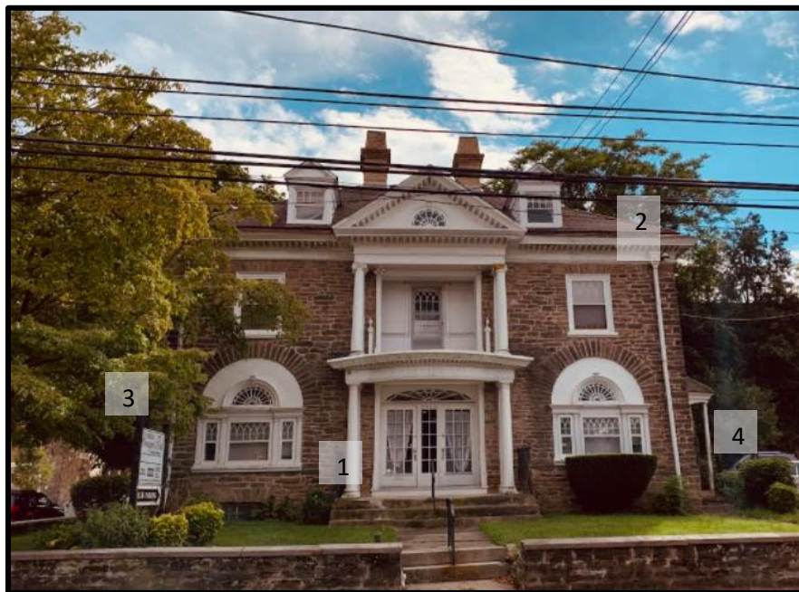
Figure 20. The primary (northeast) elevation. Source: Oscar Beisert, 2021.
