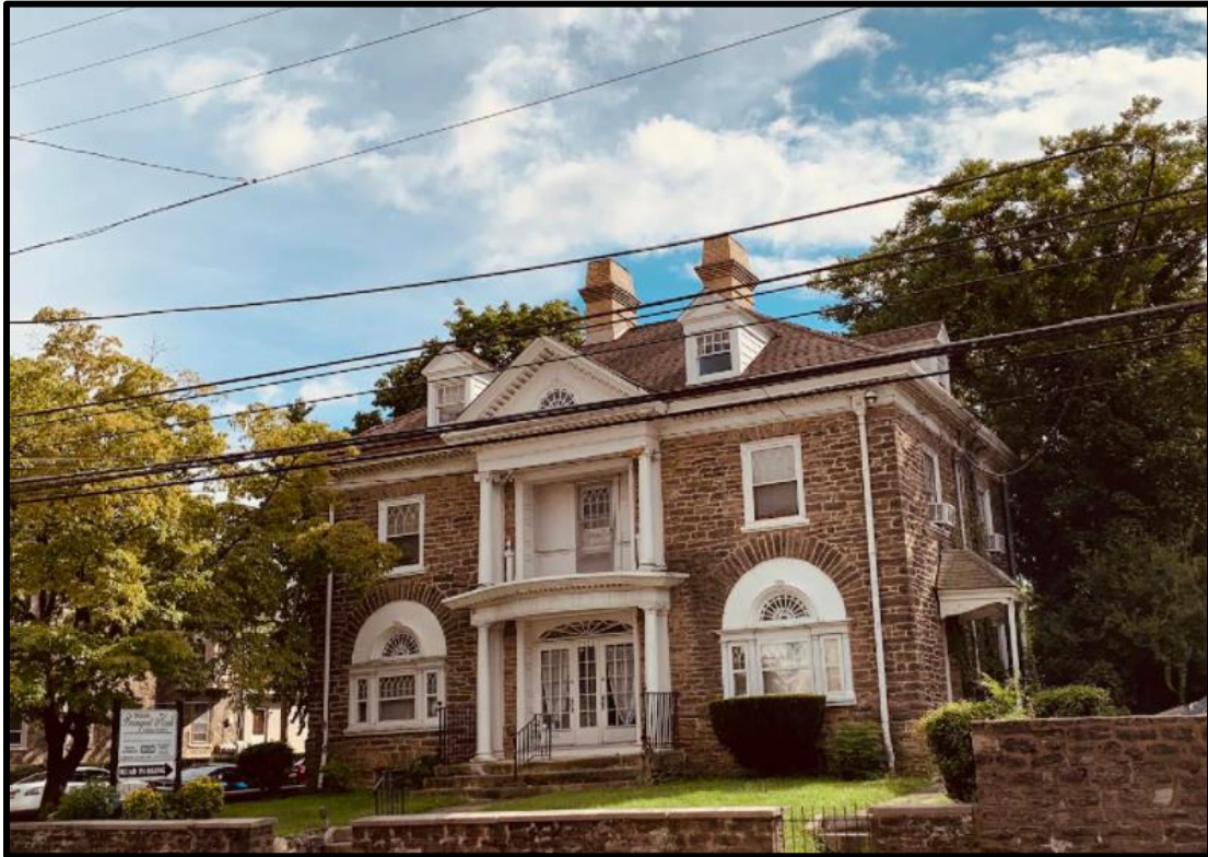
Figure 1. Looking southeast at the primary (northeast) and side (northwest) elevation of the subject house. Source: Oscar Beisert, 2021.
