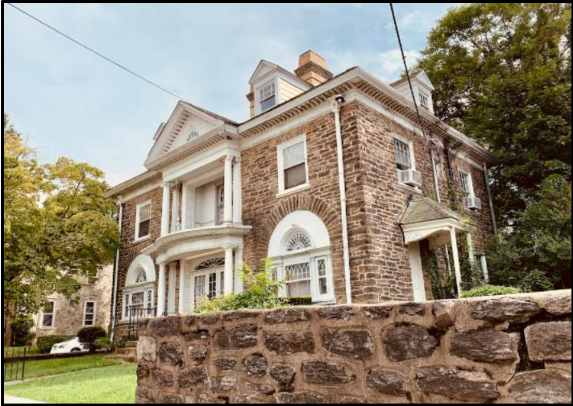
Figure 19. The primary (northeast) and northwest elevations. Source: Oscar Beisert, 2021.
