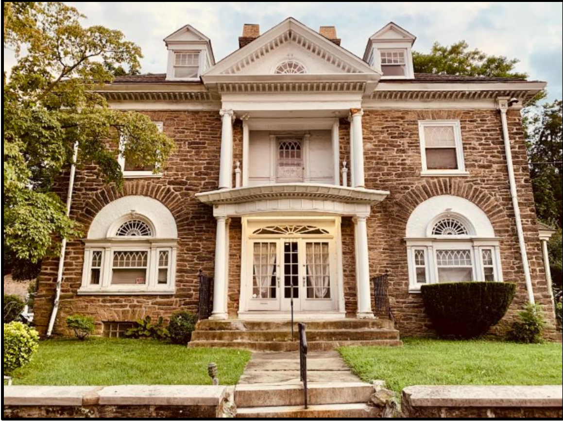
Figure 5. The primary (northeast) elevation. Source: Oscar Beisert, 2021.
