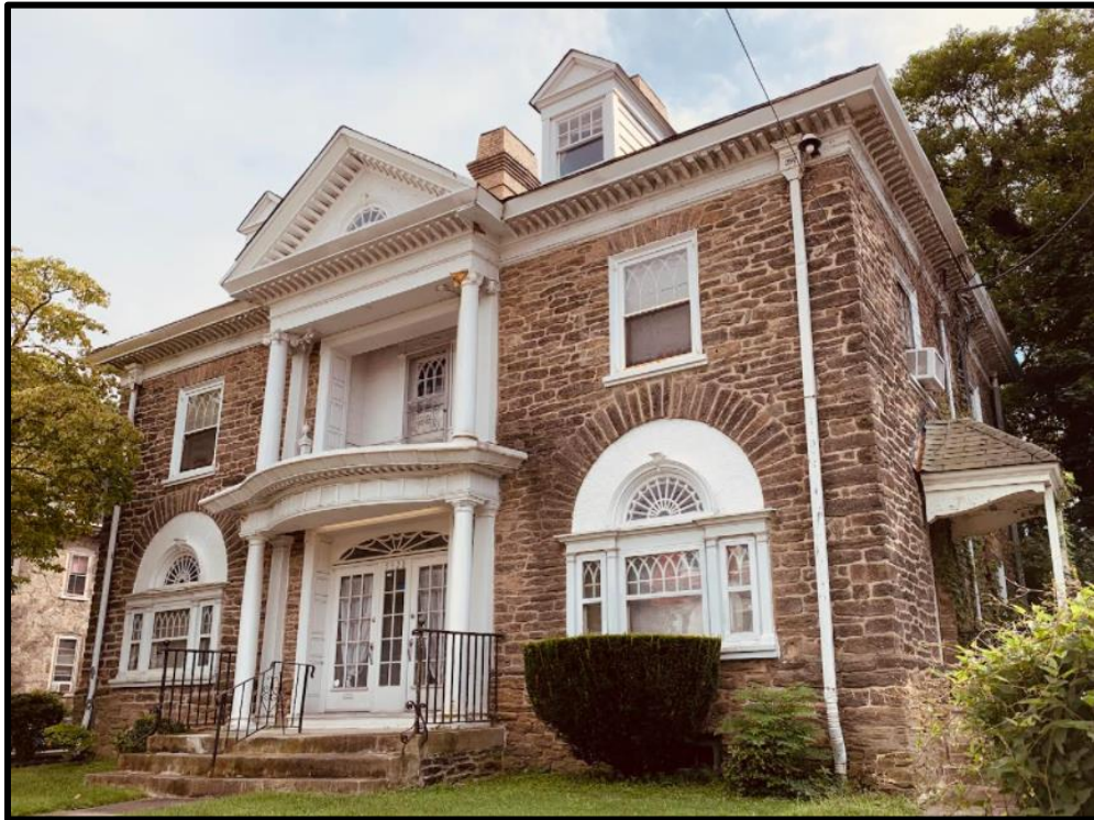
Figure 6. The primary (northeast) and northwest elevations. Source: Oscar Beisert, 2021.
