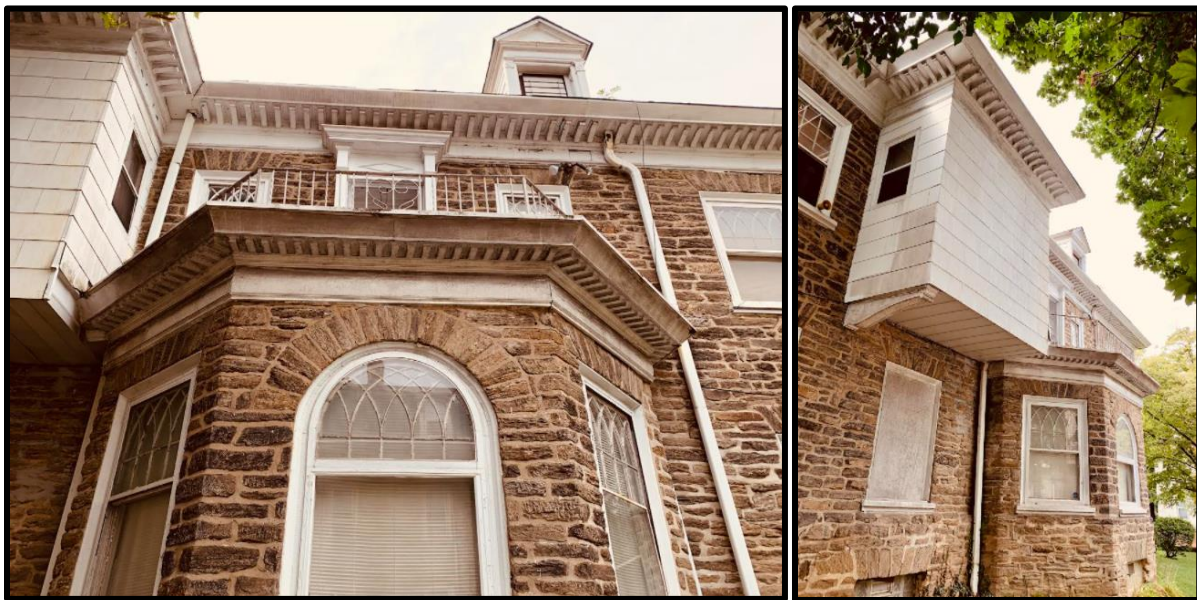
Figure 10. Left: Details of the southeast elevation. Figure 11. Right: Details of southeast elevation, including the second-story bay window and the first-story oriel window. Source: Oscar Beisert, 2021.
