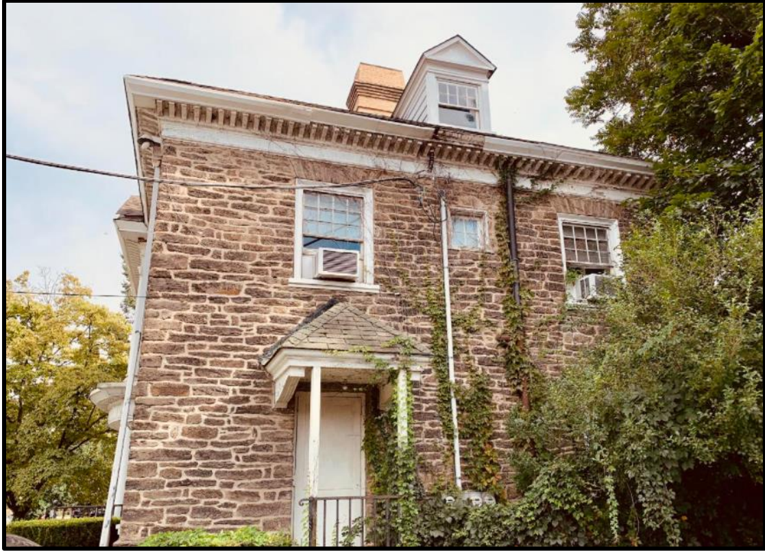
Figure 13. The northwest elevation, showing the office entrance. Source: Oscar Beisert, 2021.
