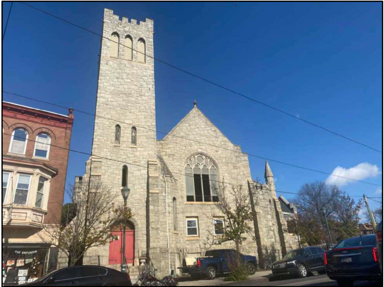
Figure 5: View north of the south elevation of Emmanuel Christian Church at 5001 Baltimore Avenue. Source: Kelly E. Wiles, November 2022.
