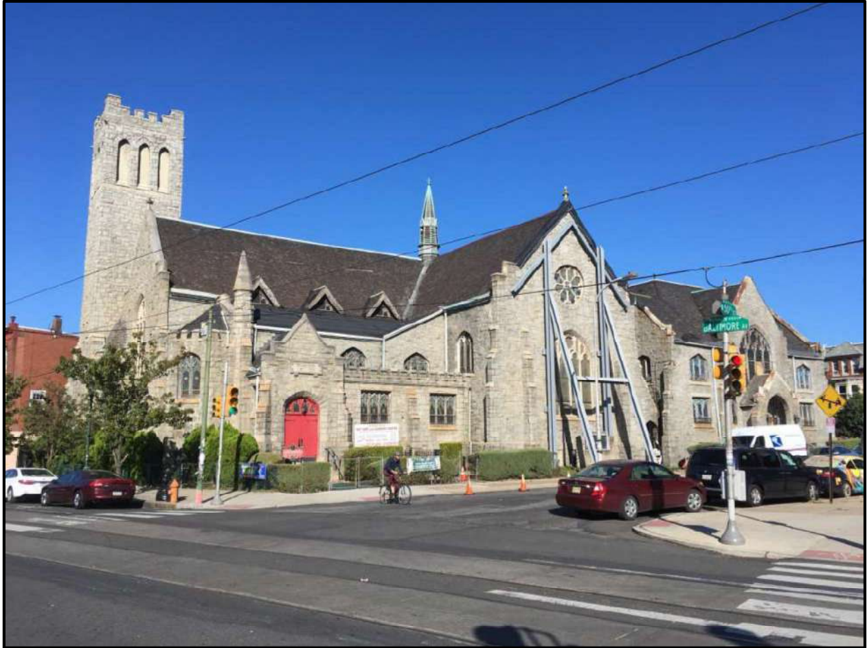
Figure 8: View northwest of the east elevation of the former Hickman Temple AME Church at 5001 Baltimore Avenue. Source: Jenny Loustau, October 2019. Note the original stained glass still intact.
