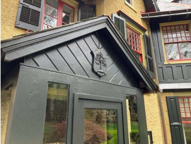
Figure 8: Detail of the entry vestibule showing the firemark. Distinctive window treatments and exterior wood paneling are also visible. Photo by Massimo Cristofanilli.
