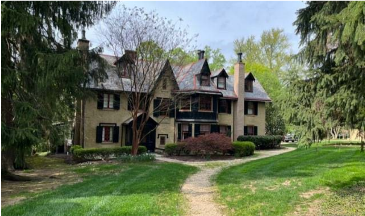
Figure 1: South elevation, photo by Massimo Cristofanilli.
