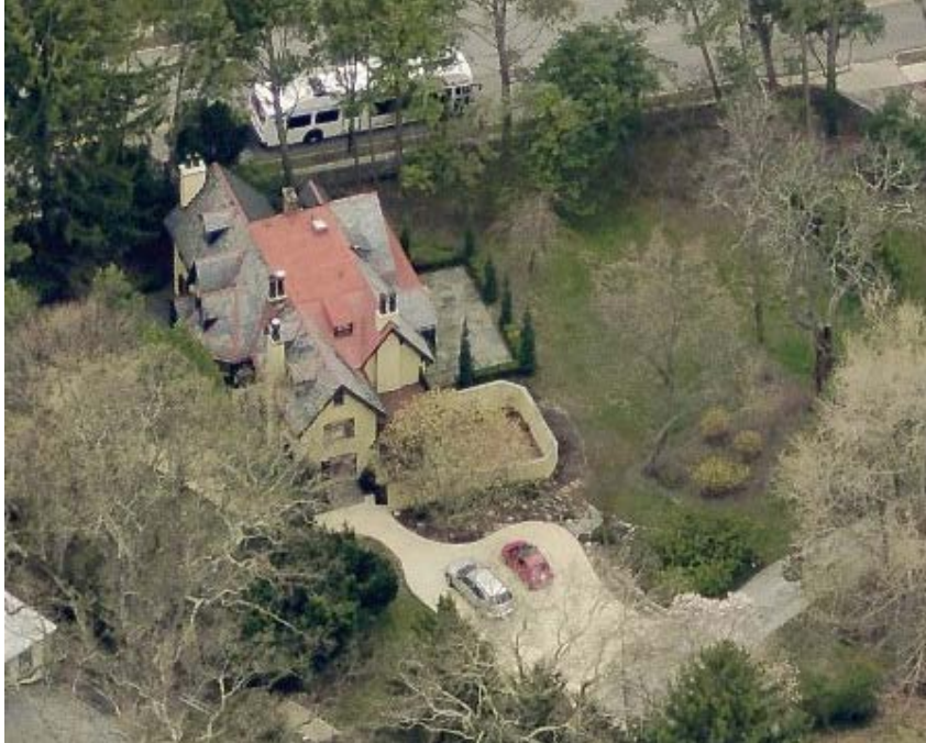
Figure 11: Aerial photo of 150 Bethlehem Pike with Bethlehem Pike at the top, showing the East elevation. Image from Pictometry.phila.gov.
