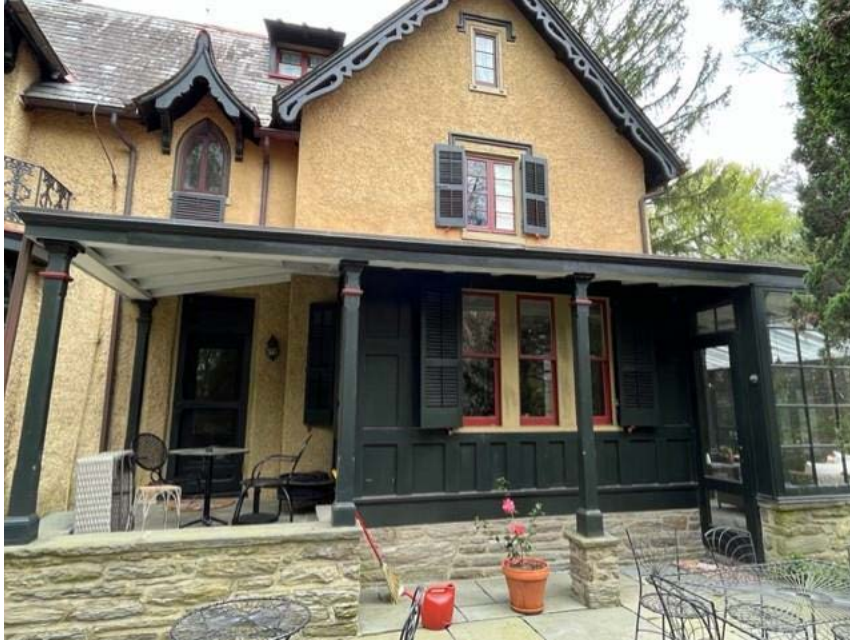
Figure 14: Detail of the North elevation, showing the sloped gable dormer, shed dormer, porch, and exterior wood paneling. Photo by Massimo Cristofanilli.
