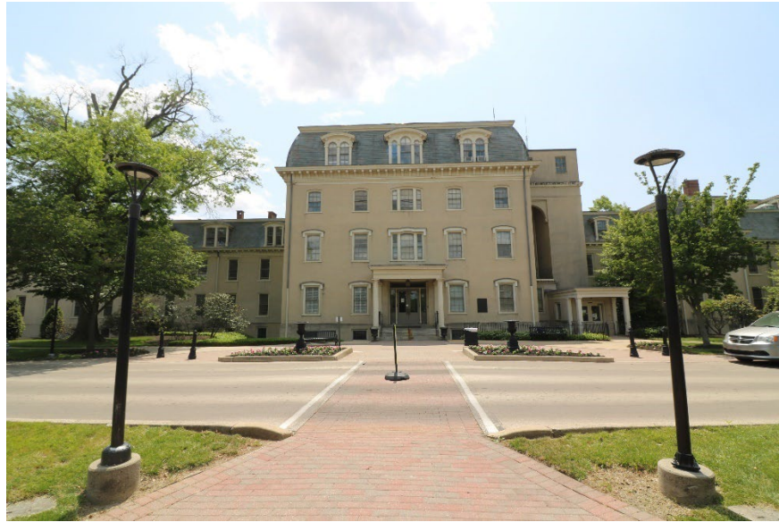
Figure 13: 2023 image of Scattergood Building illustrating the 1871 mansard roof and fourth floor addition to the main building.
