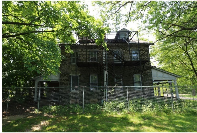
Figure 25: 2023 image highlighting metal fire escape stair along the primary, north, elevation and shed roof porch extensions from 1910
