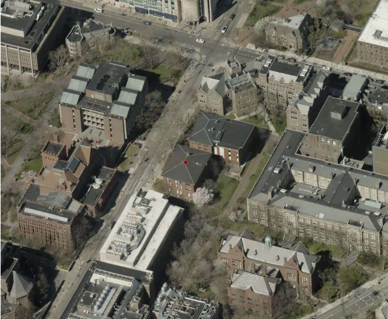
Figure 4: Aerial view of 220-60 S. 33rd Street looking north.
