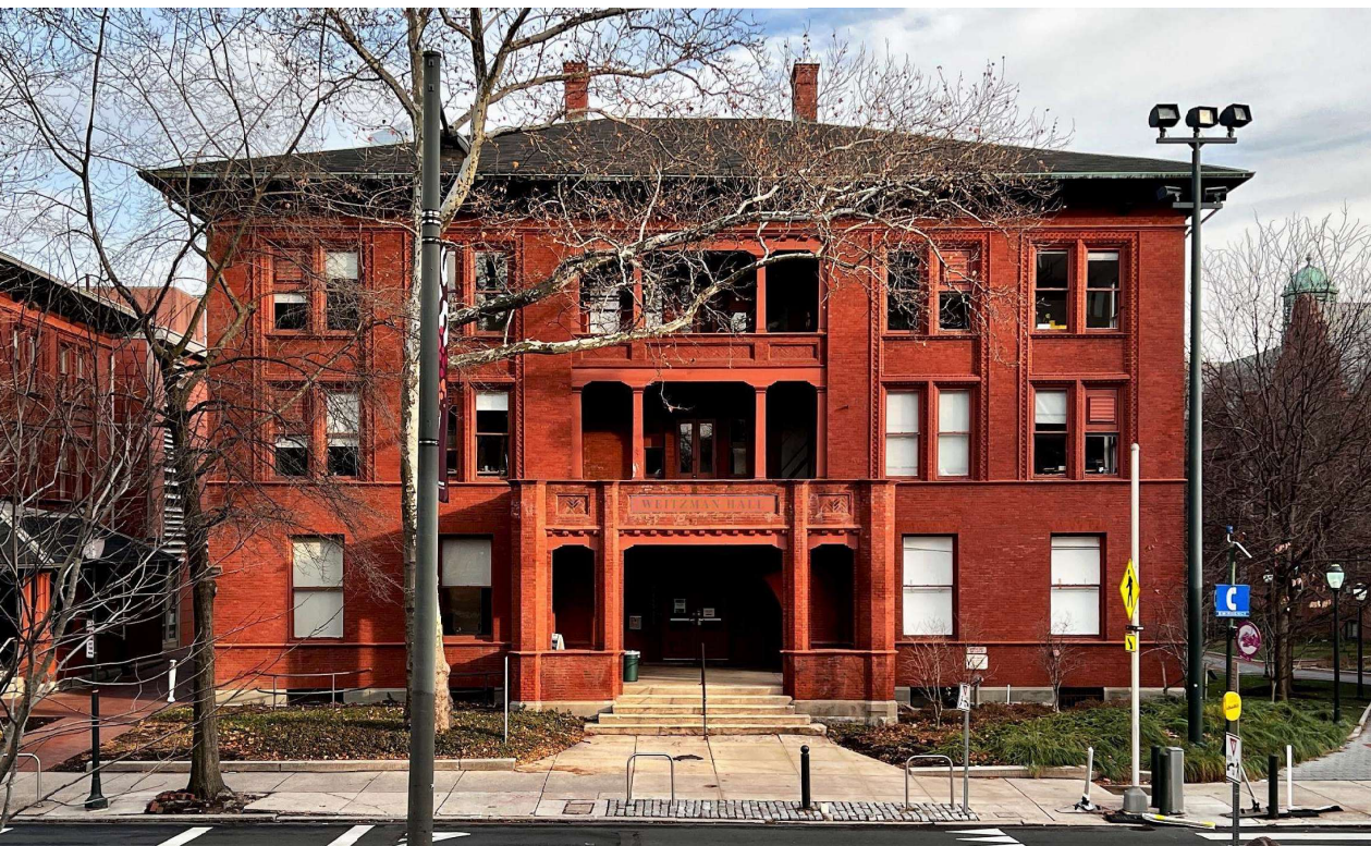
West Elevation of Stuart Weitzman Hall, December 2021
