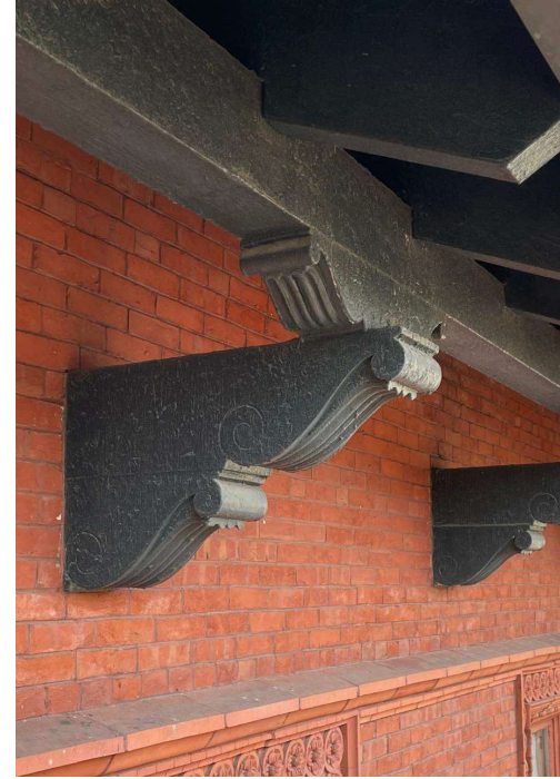
WOOD BRACKETS, SOFFIT, AND TRIM
