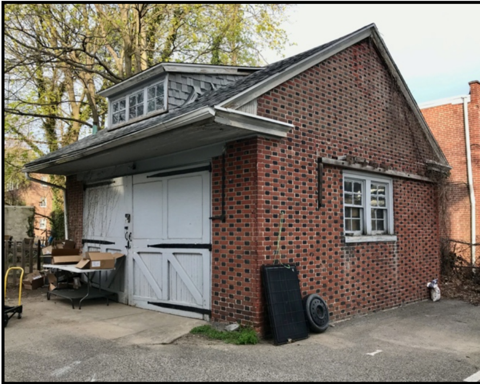
Figure 4. Top: The southwest and northwest (primary) elevations of the Garage. Figure 5. The northwest (primary) and southwest elevations of the Garage. Source: Keeping Society of Philadelphia, 2023.
