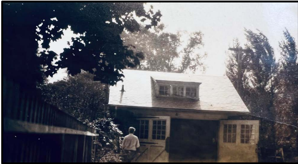
Figure 16. Top: The garage of the subject property at 150 W. Washington Lane under construction in 1919. Source: Fire Insurance Survey No. 19896, 8 May 1919, Historical Society of Pennsylvania. Figure 17. Bottom: The garage of the subject house in 1925. Source: Fire Insurance Survey No. 19896, 21 September 1925, Historical Society of Pennsylvania.
