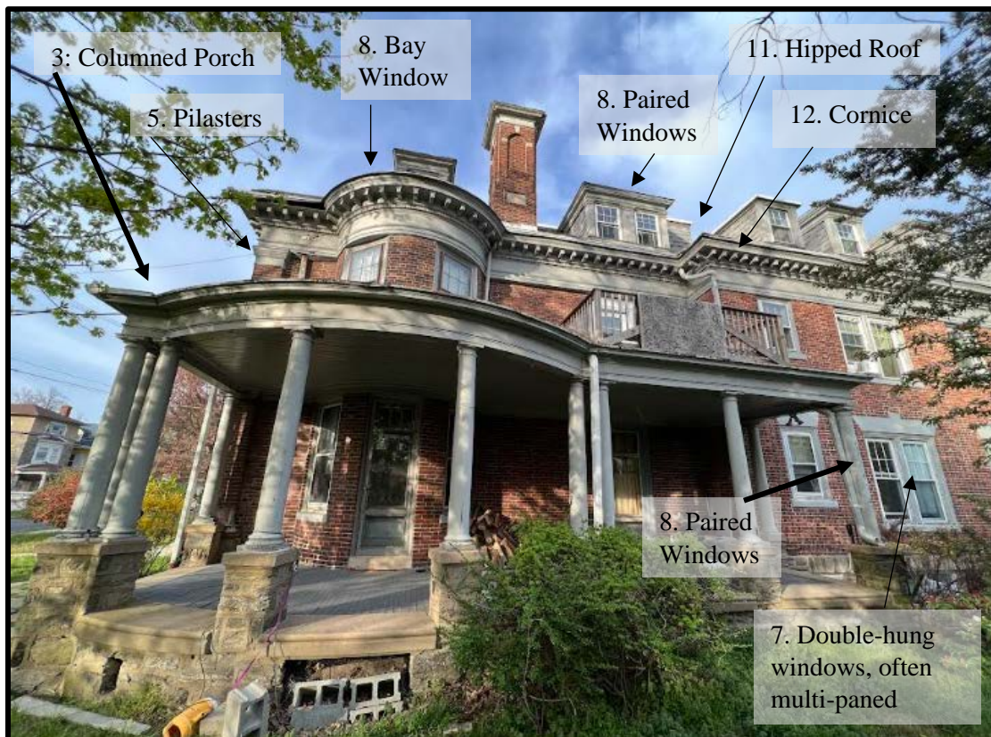
Figure 27. The southwest elevation.
