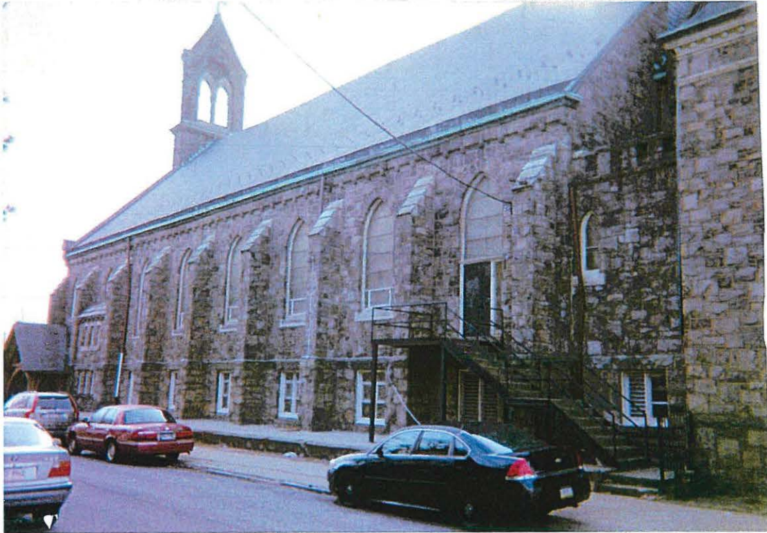
North wall on Unruh Street with buttresses between the D'Ascenzo Studio's stained glass windows.
