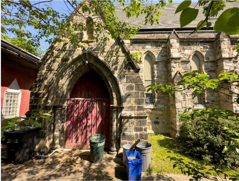
The south façade of the stone church building mimics the north façade. The long side is lit by five lancet windows which alternate with pointed buttresses. The west side of this façade has a protruding gabled vestibule with a gothic arch. The wooden plank doors are surrounded on each side by stone pilasters. Above the door is a stone niche.
