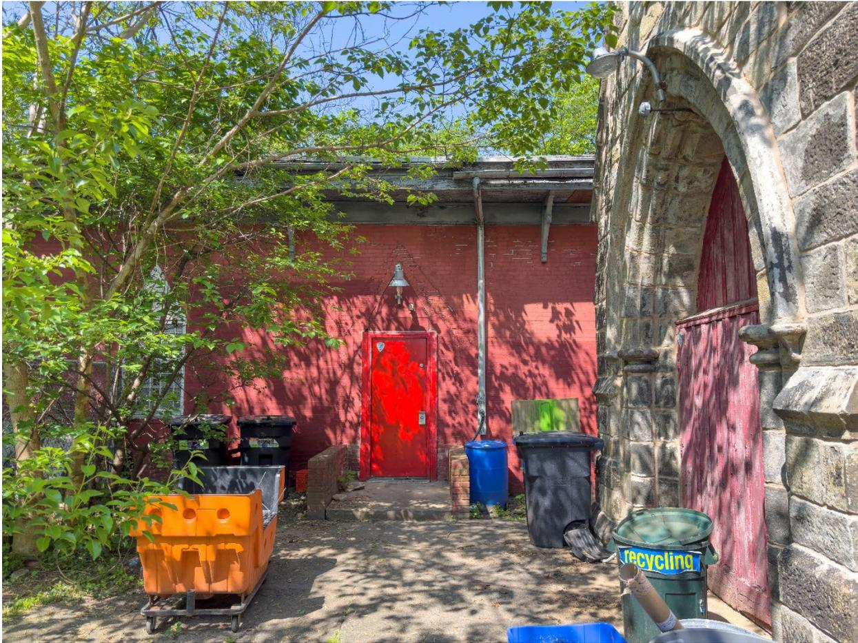
The west façade of the meeting hall is a simple red painted brick face. Above the door are remnants of what could have been an awning to shelter the door opening from the elements. The overhanging roof is decorated with wooden cornice brackets. There is a window to the left of the door with a triangular opening above, like the windows on the south façade of this Meeting Hall.
