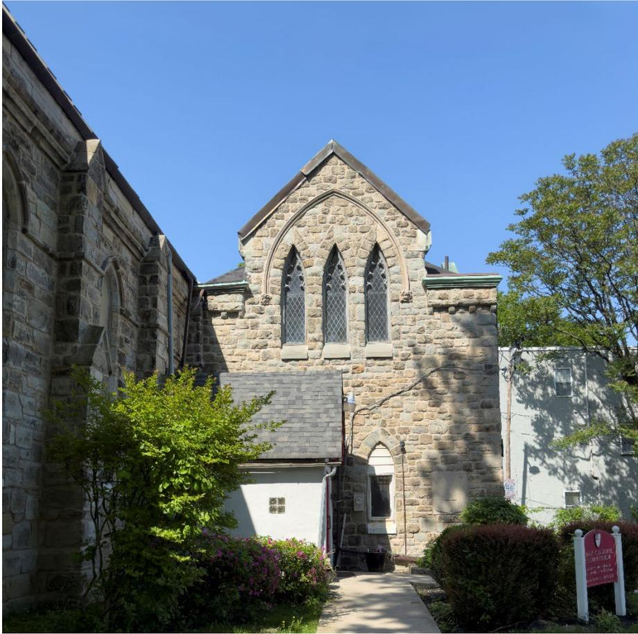
The west façade of the Parish House is clad in rough stone, matching the stone on the church, with a gabled roof. This façade is 2 bays wide and 2 ½ stories tall. A group of three pointed gothic openings of leaded glass adorn the upper section of this façade, with a gothic arched crown. At the base of the arch are stone or terracotta figures of heads surrounded by leaves.
