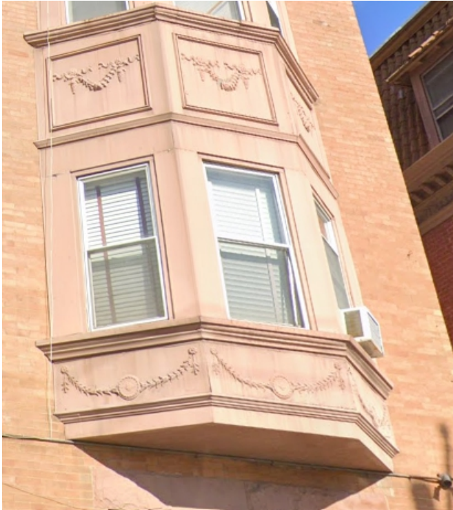
Detail of oriel and cornice bracket, Google
