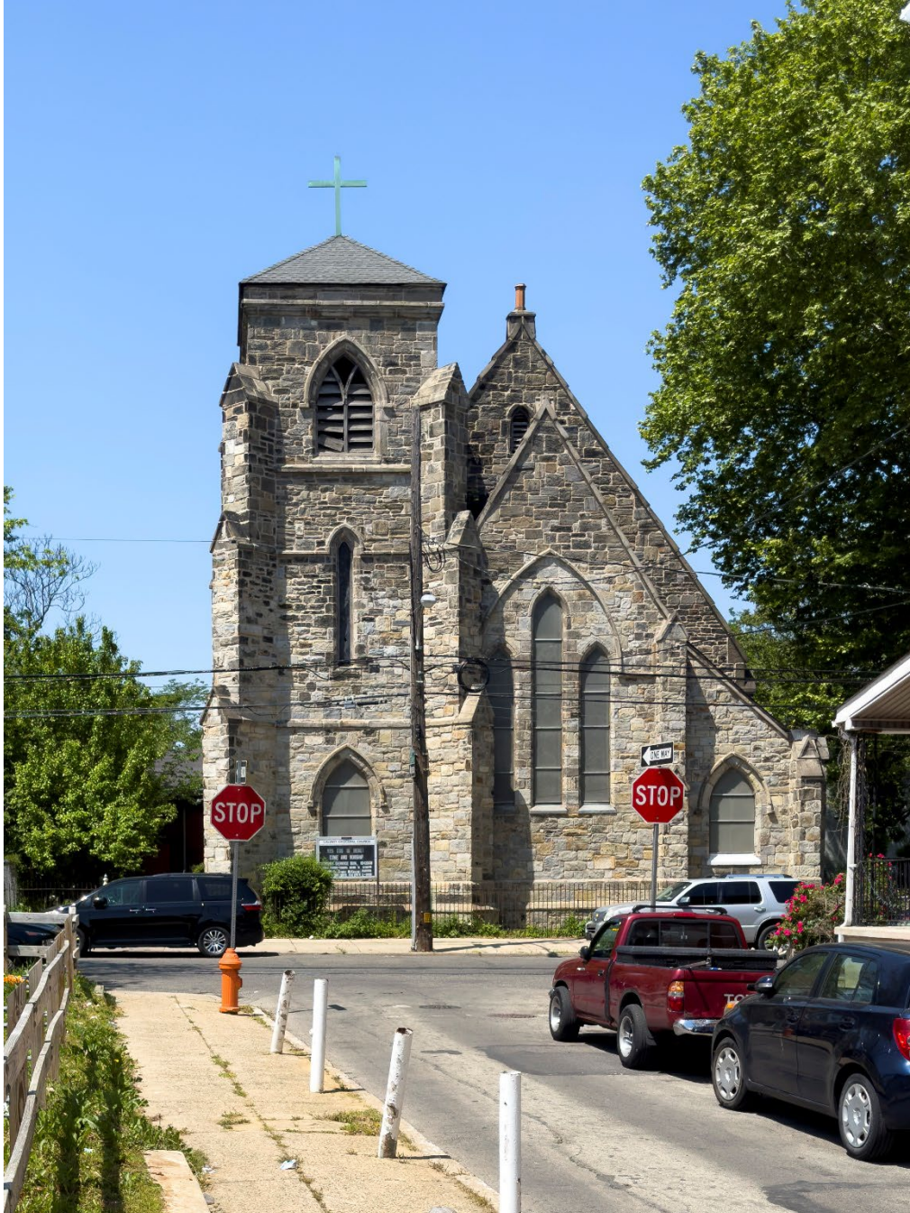
Calvary St. Augustine Episcopal Church Built originally in 1851; moved and rebuilt in 1882
