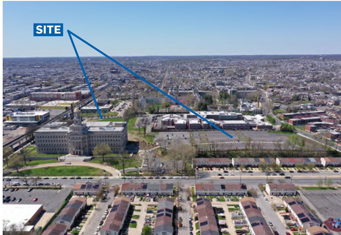
A-1: AERIAL VIEW OF SITE LOOKING WEST
