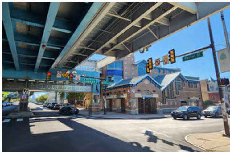
N-2: 46TH & MARKET STREETS CORNER FACING SOUTHEAST
