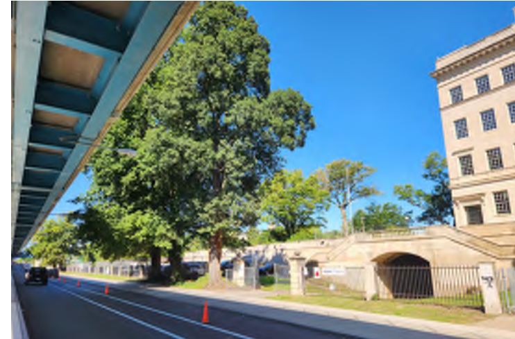
S-3: MARKET ST FACING NORTHWEST TOWARDS SITE'S FUTURE THROUGH-BLOCK CONNECTION ENTRY AT MARKET STREET
