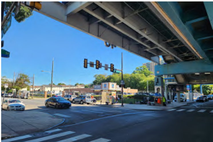
N-1: 46TH & MARKET STREETS CORNER FACING NORTHEAST
