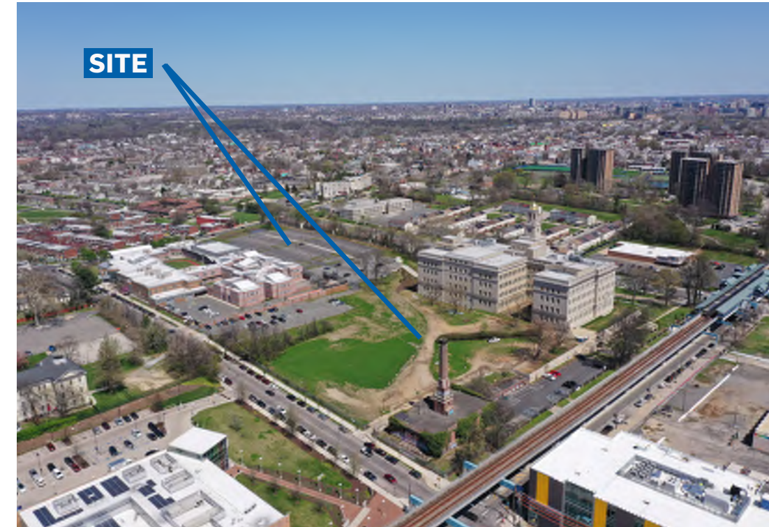
A-4: AERIAL VIEW OF SITE LOOKING NORTHEAST
