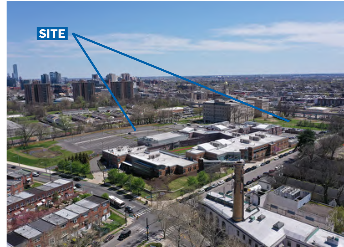
A-6: AERIAL VIEW OF SITE LOOKING SOUTHEAST
