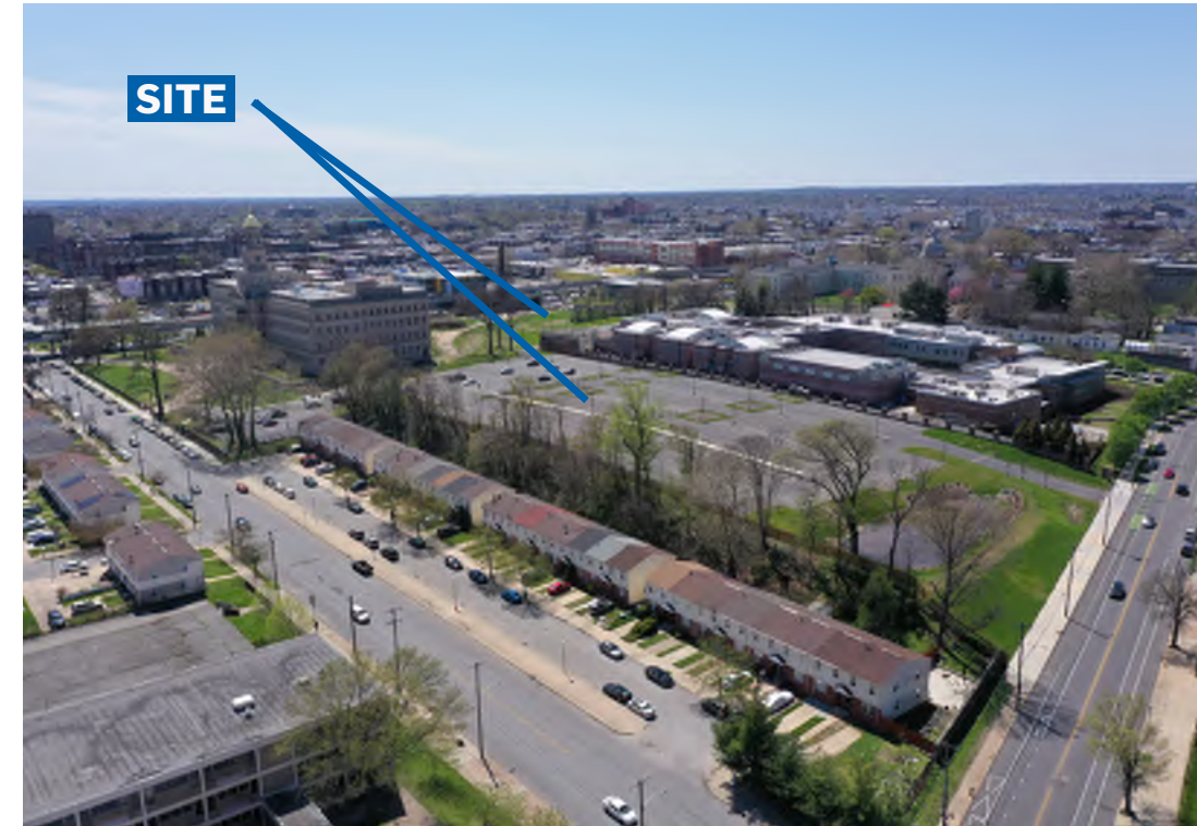
A-8: AERIAL VIEW OF SITE LOOKING SOUTHWEST
