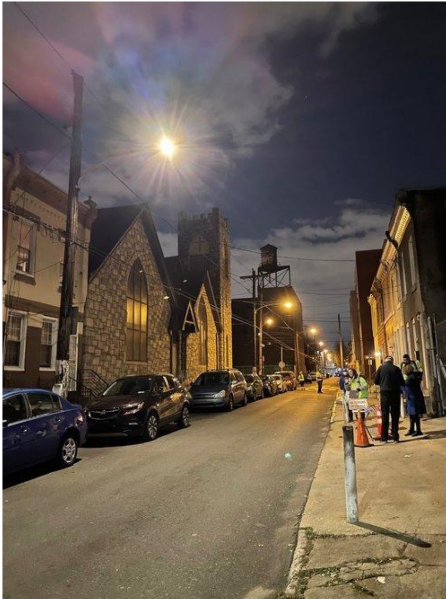
FIGURE 2 THE CITY OF PHILADELPHIA AND THE PHILADELPHIA ENERGY AUTHORITY (PEA), IN PARTNERSHIP WITH AMERESCO, INC., HAVE LAUNCHED TRIAL INSTALLATIONS FOR THE PHILLY STREETLIGHT IMPROVEMENT PROJECT (PSIP)
