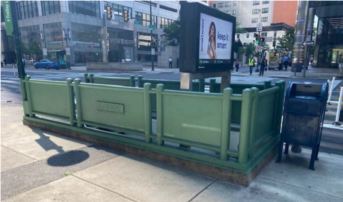
Figure 2: North and west sides of the Northwest corner entrance to the 19 th and Market Street trolley, 2022.
