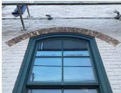
B EXISTING WINDOWS MATERIAL: WOOD COLOR: TBD, PT TO MATCH NEW WINDOWS OPERATION: DOUBLE HUNG
