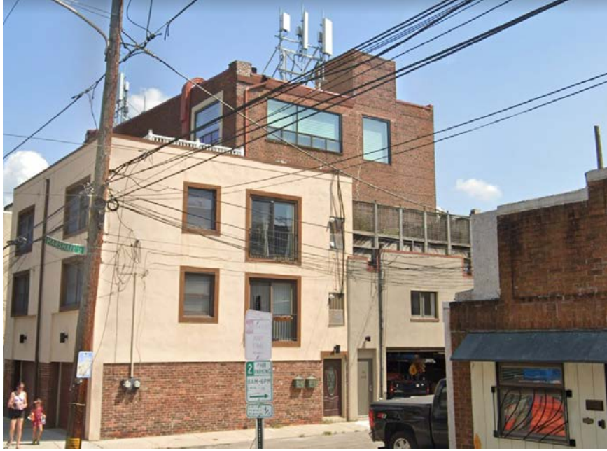
Figure 7. View of rear from Bainbridge Street, August 2022. Only the upper floors with telecommunications equipment are visible. Source: Google.
