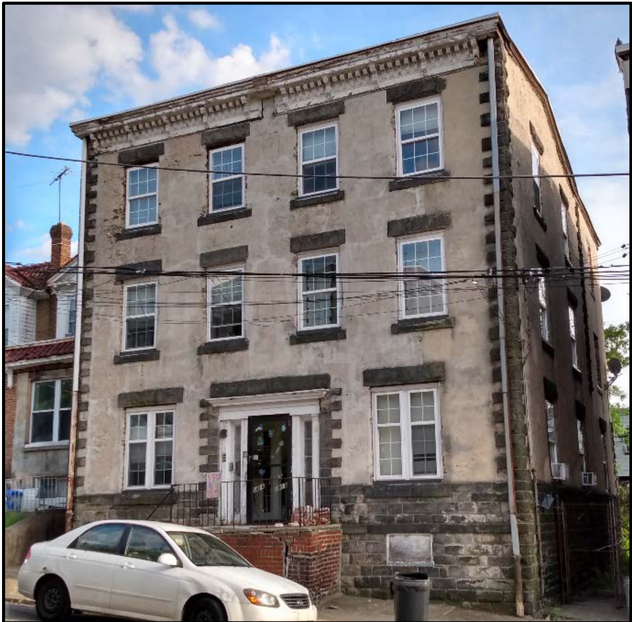
Figure 8: North (front) façade of 3414-16 W. Westmoreland Street.
