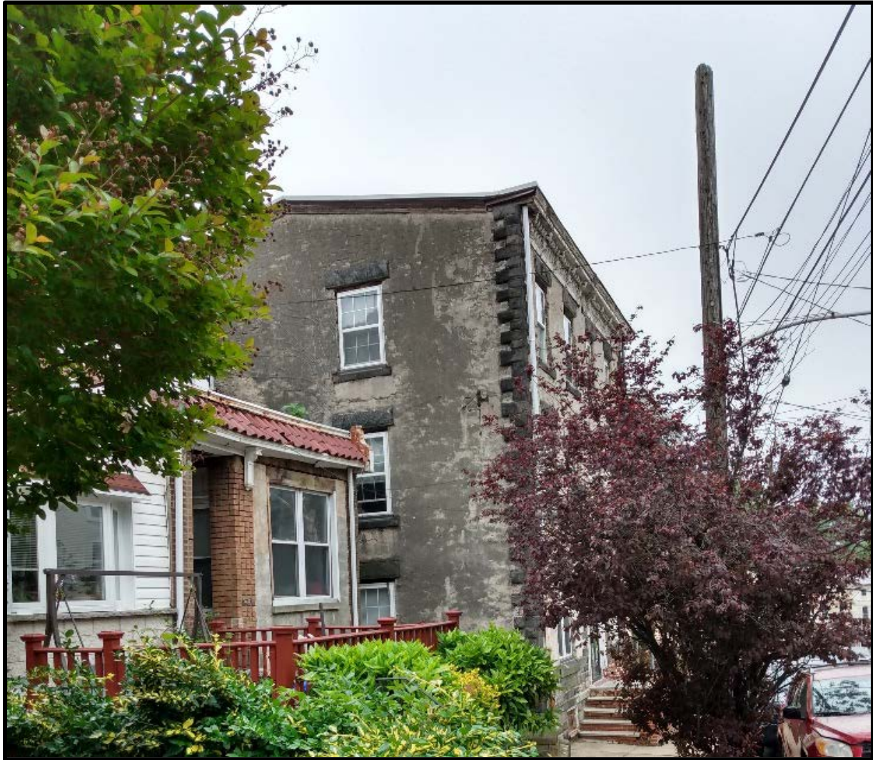
Figure 9: 3414-16 W. Westmoreland Street east elevation.
