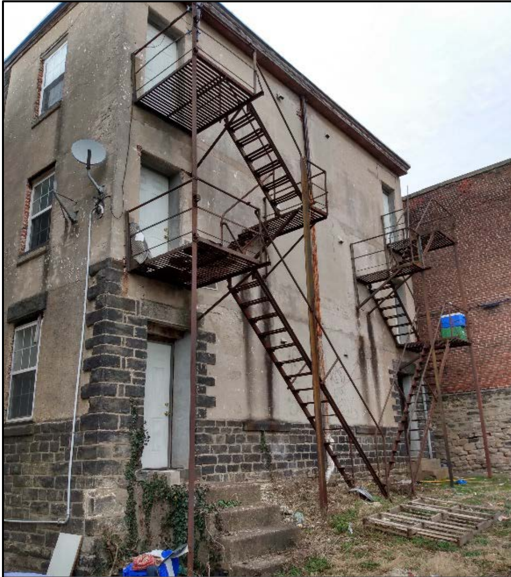
Figure 10: Rear of 3414-16 W. Westmoreland Street.
