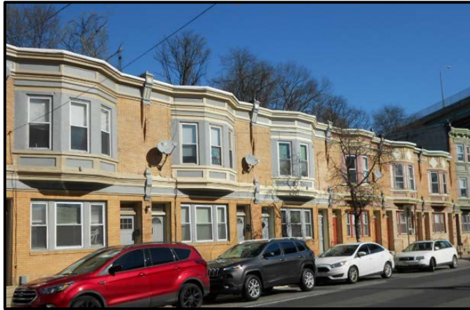
Figure 14: Houses built by John Dobson c. 1900, 4200 block of Ridge Avenue. Built as three-stories, later shortened for unknown reason. Courtesy N. Pontone
