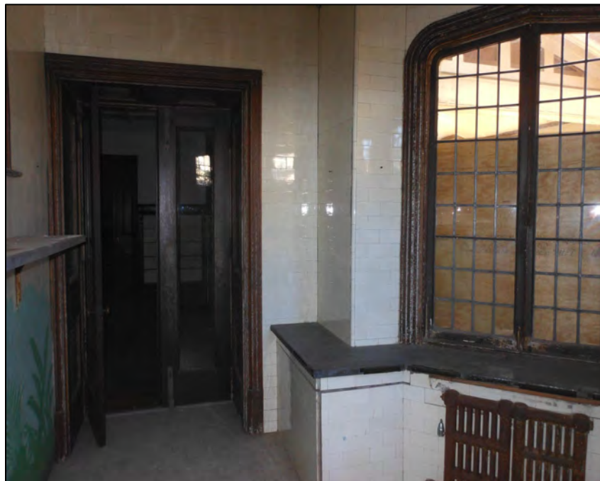
Photo 20. Tiled first floor solarium.
