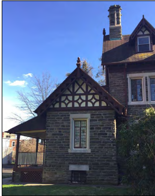
Photo 11. Northwest (side) elevation of the rear wing, facing southeast.
