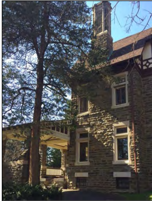
Photo 8. Southeast side elevation looking to the porte cochere, facing west.
