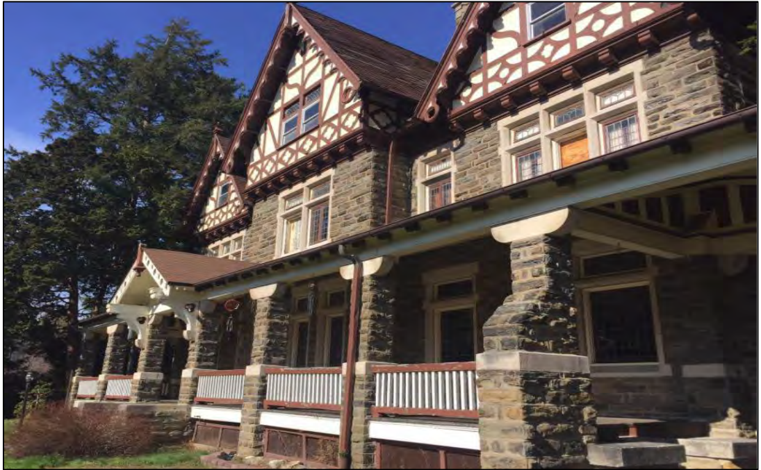
Photo 5. Front façade porch details, southwest elevation, facing north.
