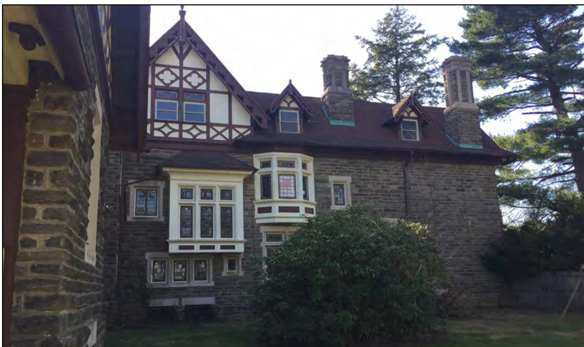
Photo 13. Northeast (rear) elevation of the main block, facing southwest.
