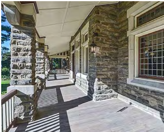
Photo 7. Front porch detail, facing north.
