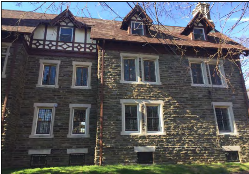
Photo 9. Southeast side elevation, facing north.
