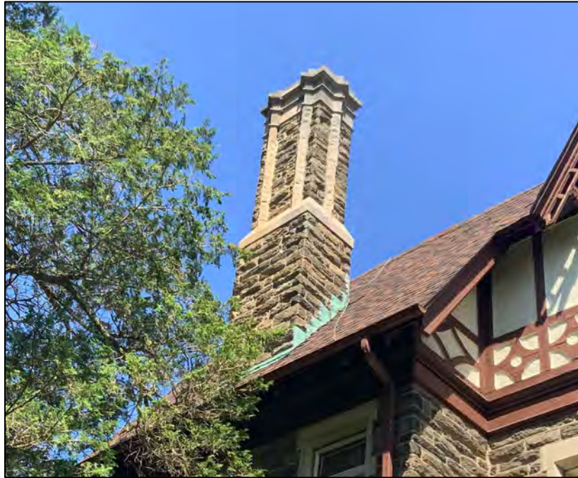
Photo 16. Decorative chimney detail, facing northwest.
