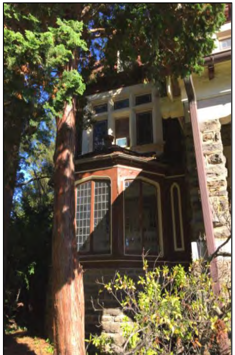
Photo 6. Front elevation bay window to the north of the porch, facing northeast.
