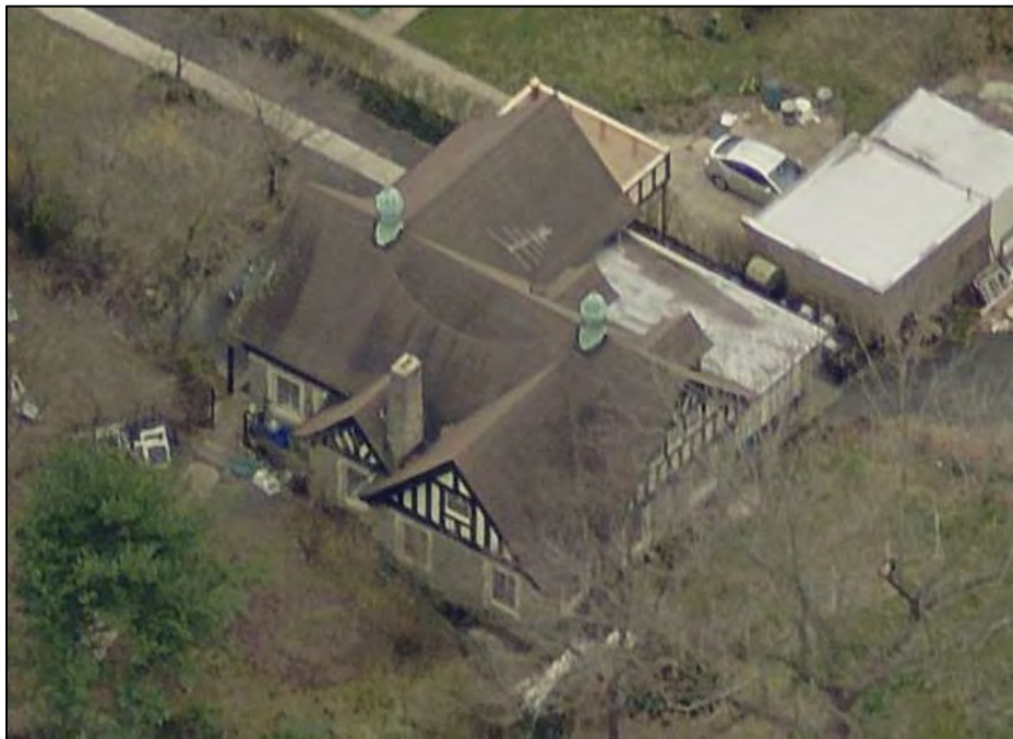
Figure 3. Carriage house and garage looking south (Bing Birdseye View).
