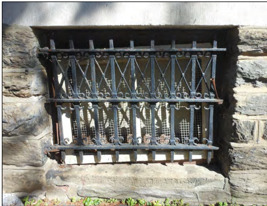
Photo 15. Basement window ironwork, facing northwest.
