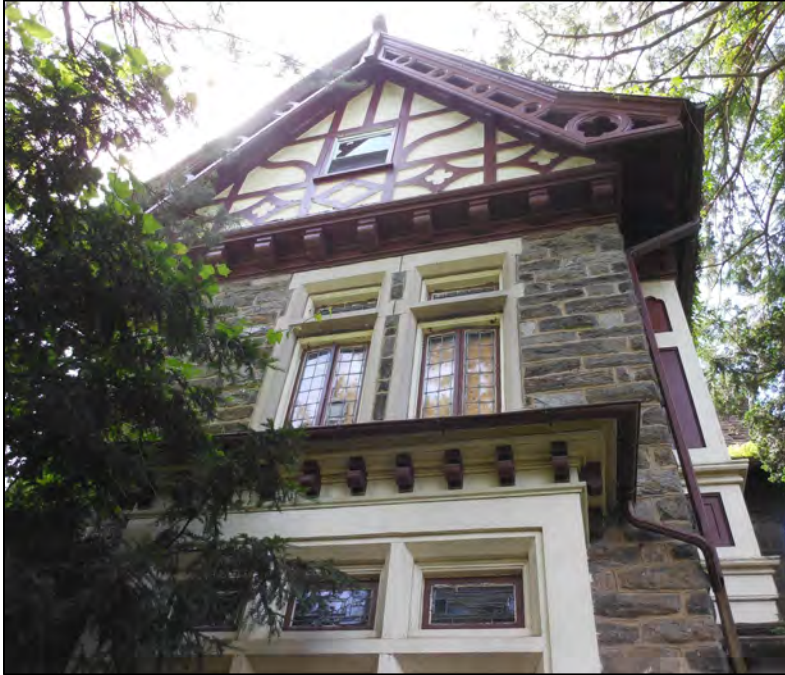
Photo 14. Northwest (side) Elevation, facing southeast.
