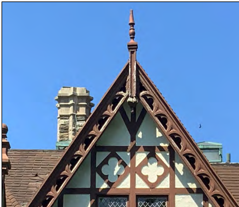
Photo 17. Carved bargeboards and finial with chimney and skylight beyond, facing southwest.
