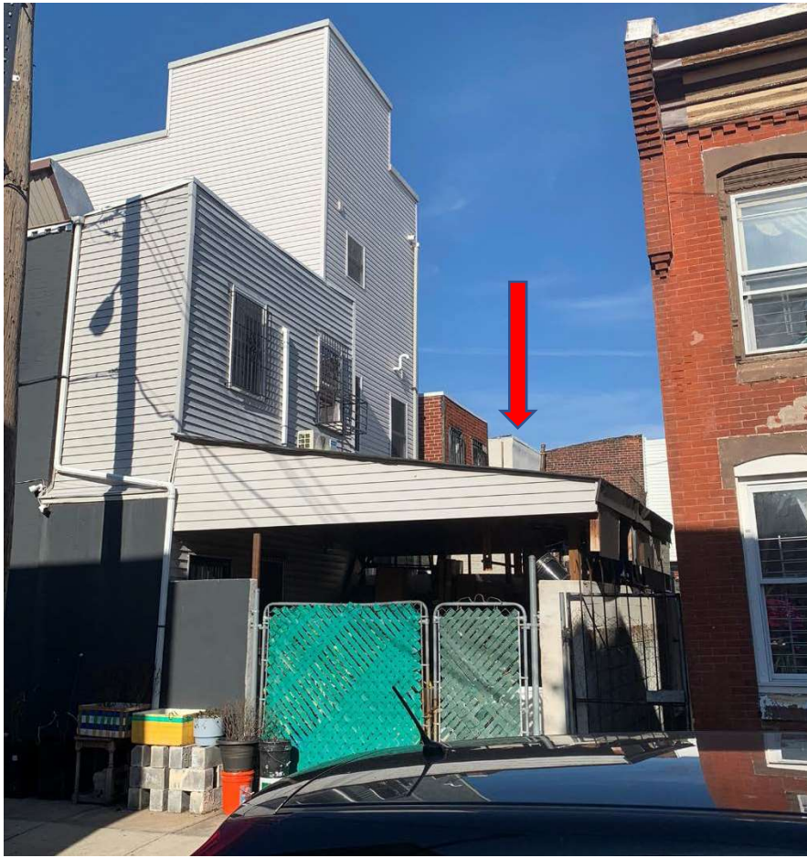
Figure 4. View of rear from Daly Street, December 2022. Only a very small section is visible, in white.
