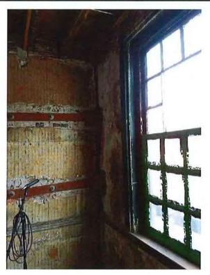
Photo 7 - View of Roof Framing Unit 212 (North Elevation) Not Tied into Exterior Wall
