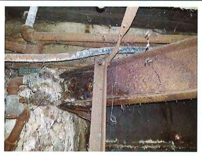
Photo 2 - Joist Deterioration in Unit 208 (Basement)
