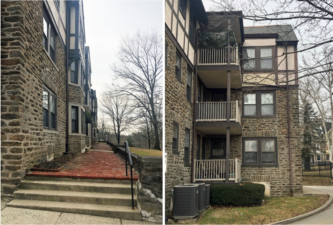
Images: Detail of front entry terrace on West Johnson Street; Detail of porch balconies; Sherman Aronson 2023-01
