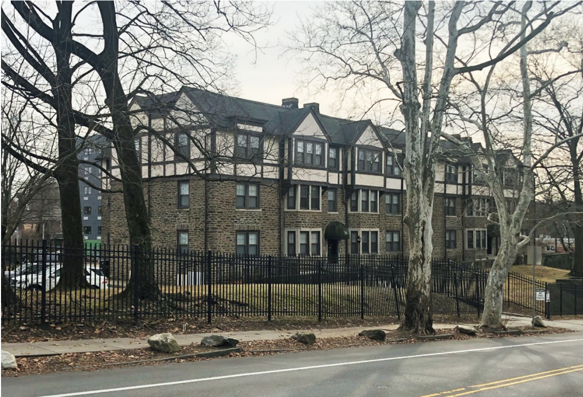
Image: View of West Johnson Street Façade from the northwest, Sherman Aronson 2023-01
