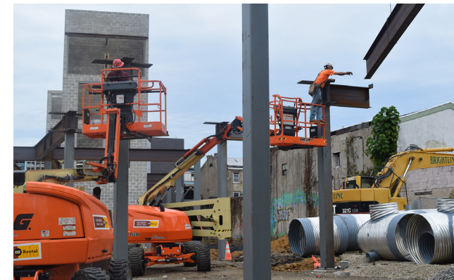
Construction of senior housing complex, Frankford
