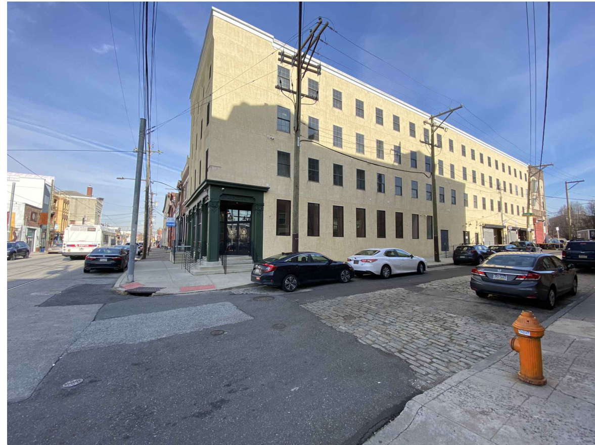
VIEW OF WILDEY ST SIDEWALK & STREET
