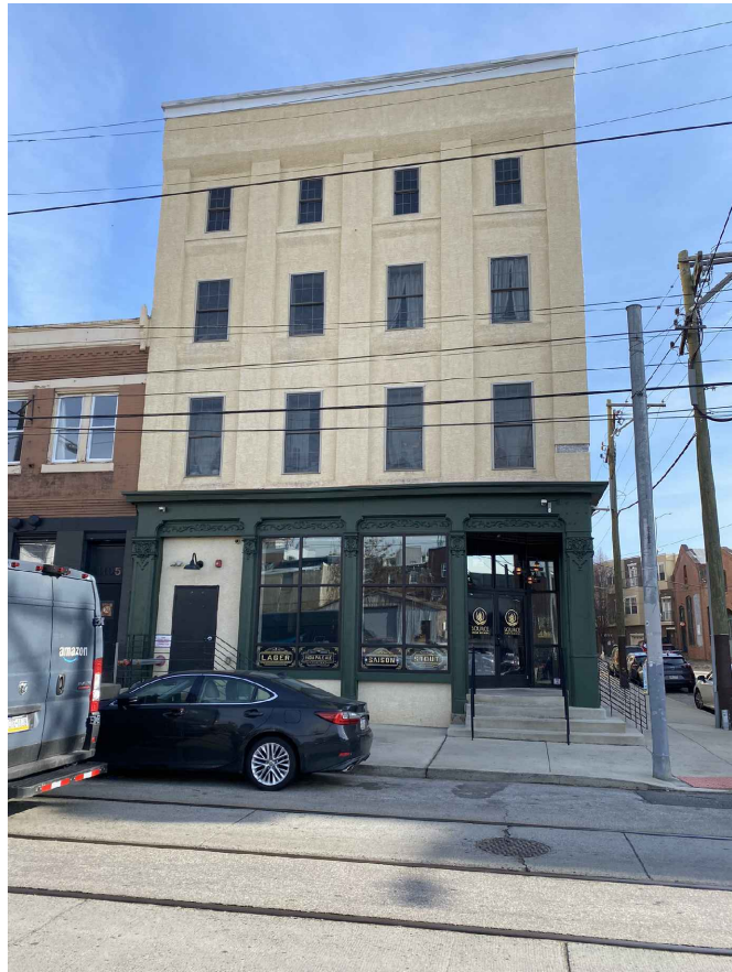
VIEW OF FRANKFORD AVE SIDEWALK & STREET
