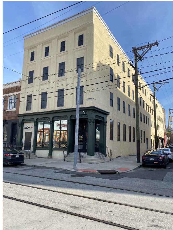
VIEW OF INTERSECTION SIDEWALK & STREET
