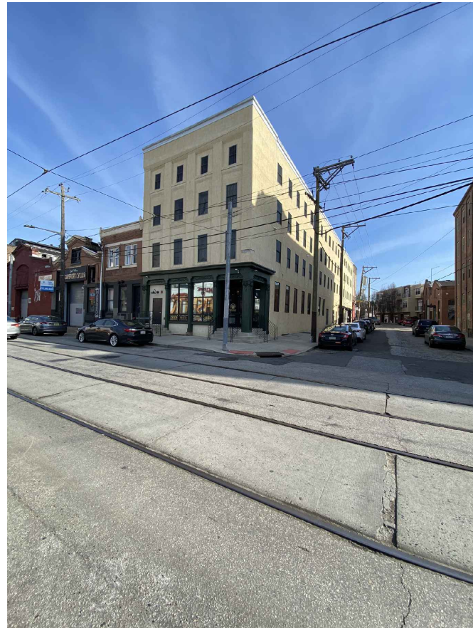
VIEW OF INTERSECTION SIDEWALK & STREET
