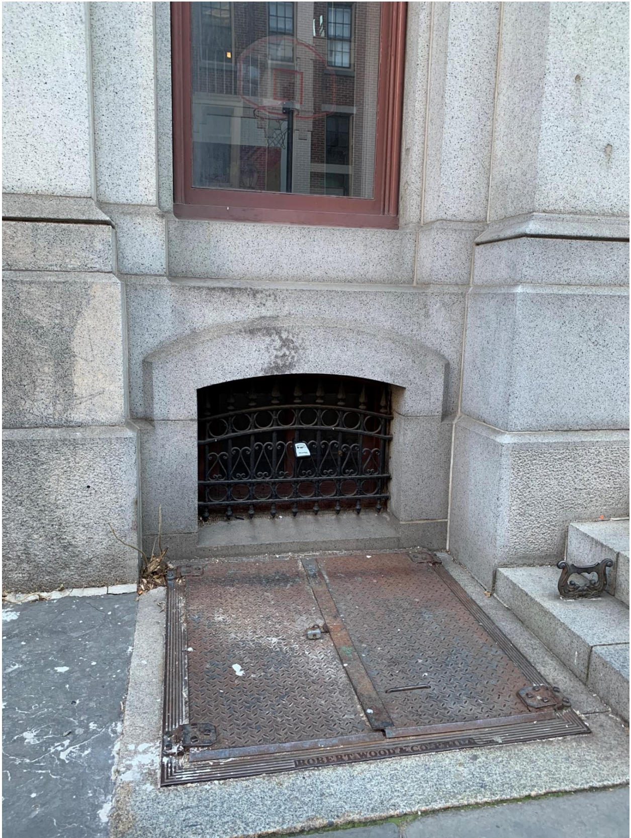
Figure 2. Existing conditions, March 2023.
