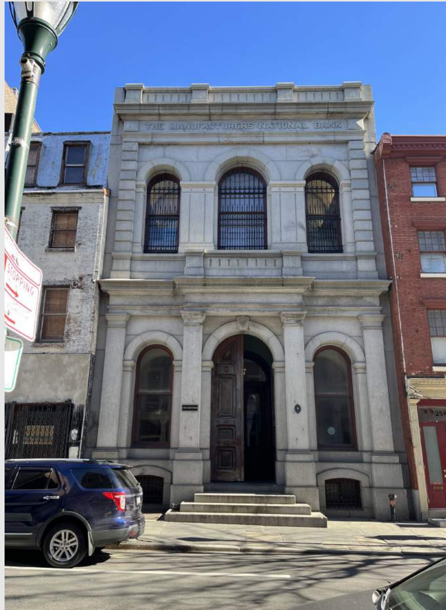
NORTH 3RD STREET FACADE
