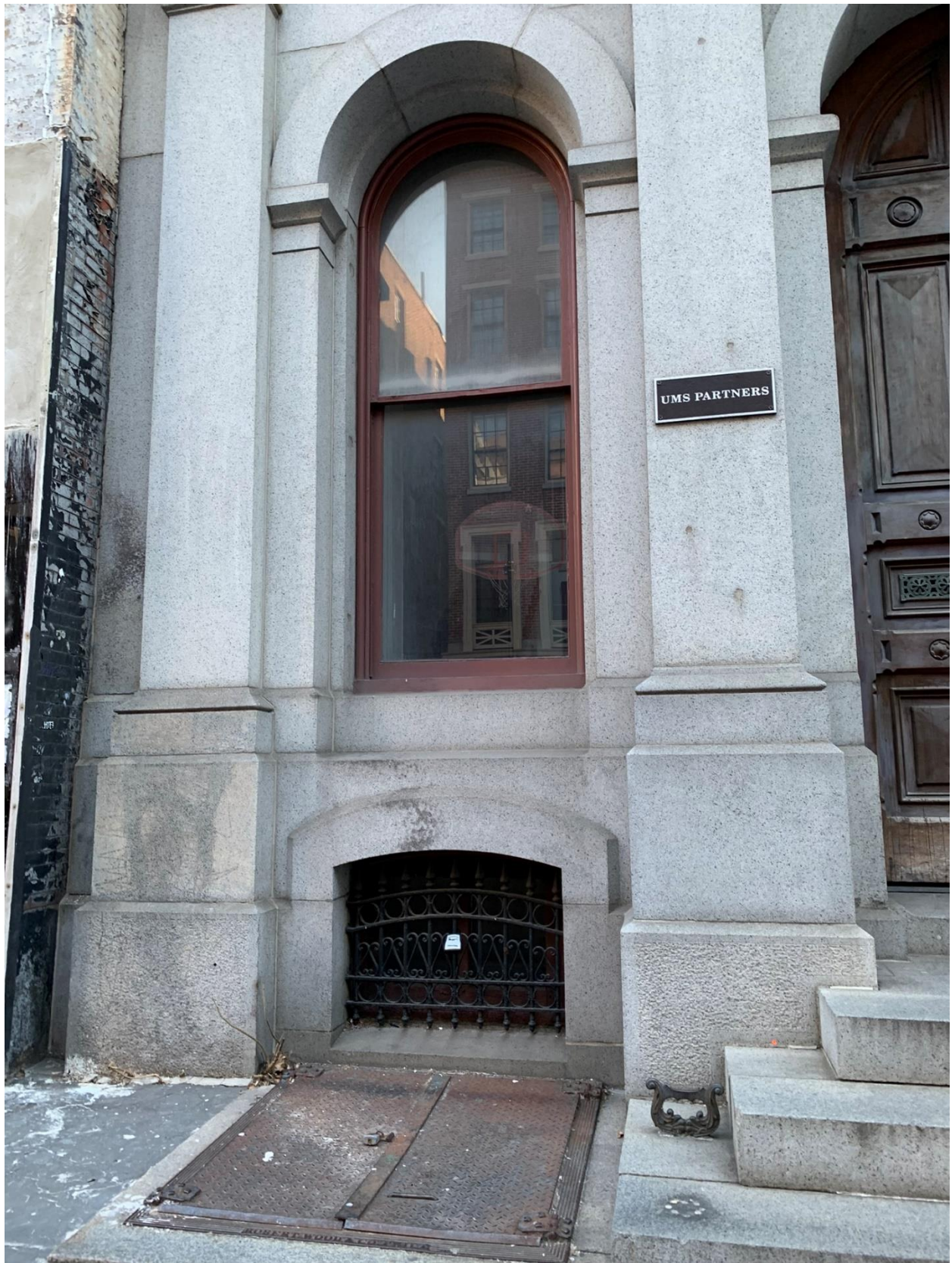
Figure 1. Existing conditions, March 2023.
