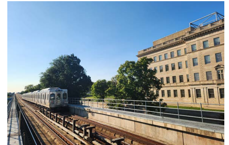
S-24: 46TH ST STATION PLATFORM FACING NORTHWEST AT SITE
