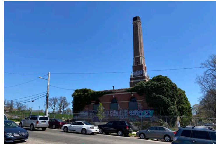
S-6: 48TH & MARKET ST CORNER FACING EAST AT SITE
