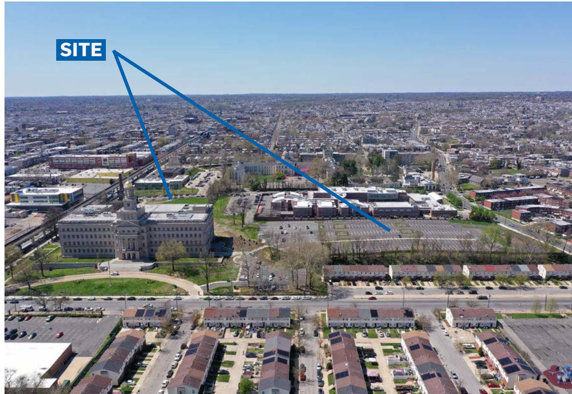
A-1: AERIAL VIEW OF SITE LOOKING WEST
