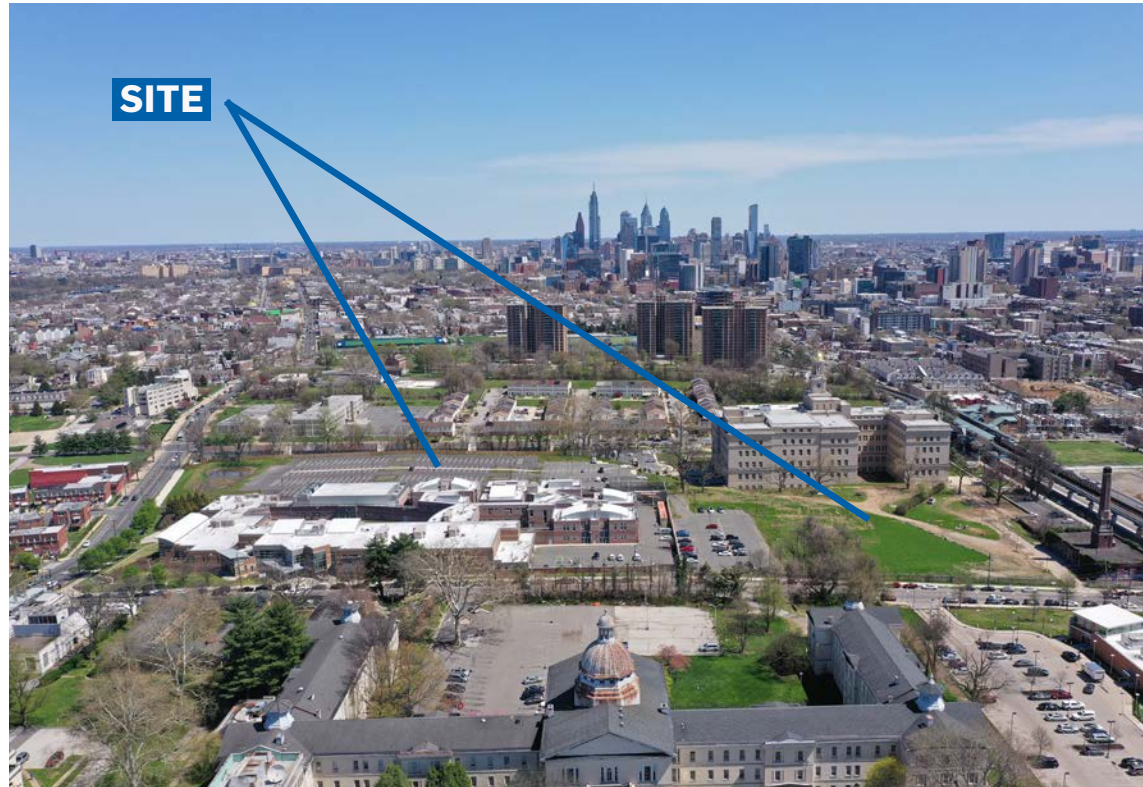
A-5: AERIAL VIEW OF SITE LOOKING EAST
