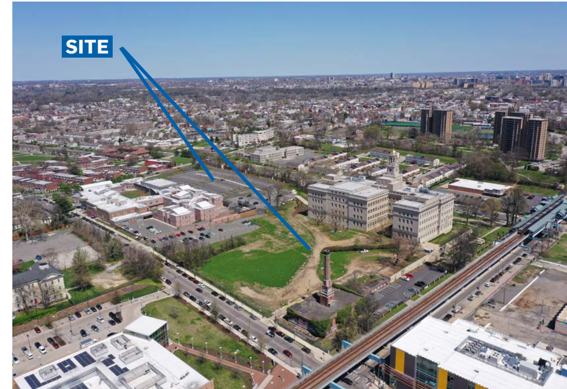
A-4: AERIAL VIEW OF SITE LOOKING NORTHEAST
