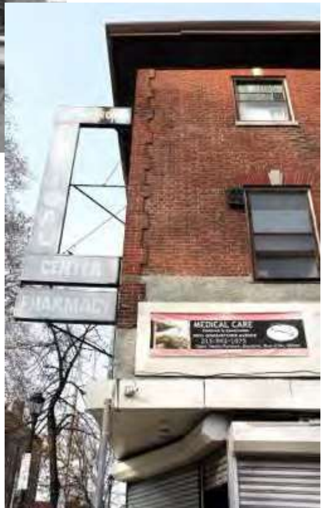
Figure 7: The southern corner of the building shows layers of modifications, including the mid-century sign and stucco covering up scars from the cornice which once ran along the first floor.
