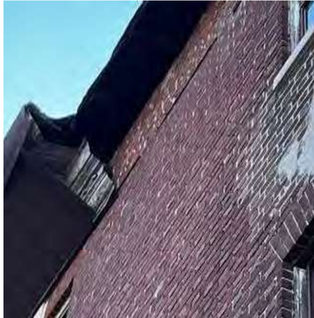
Figure 3: A portion of previous cornice is visible beneath the vinyl cornice.
