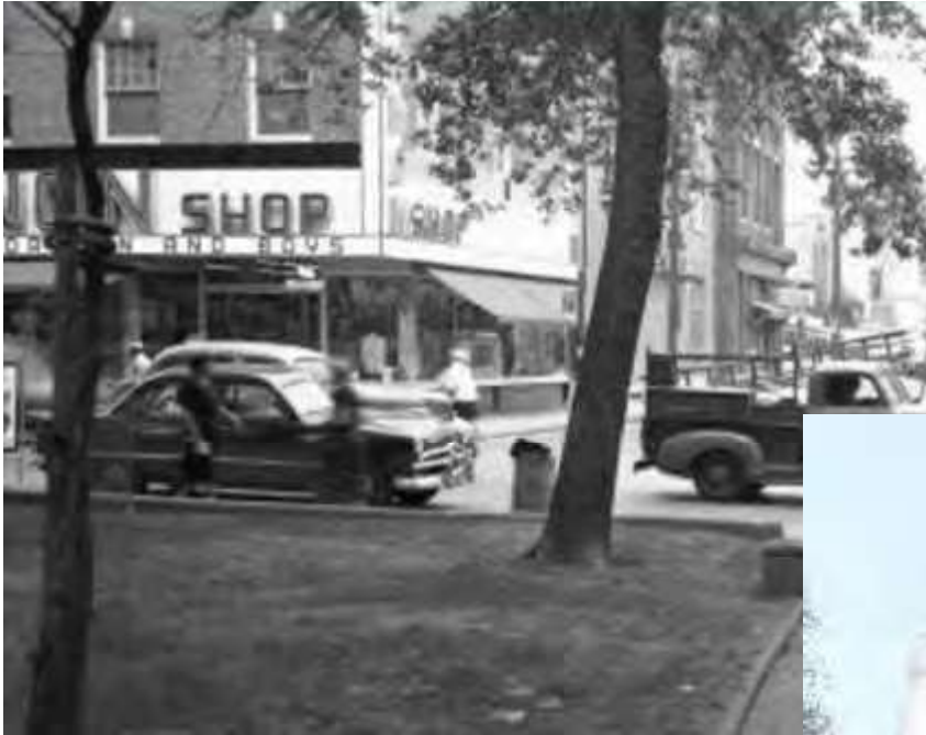
Figure 6: A photo from 1951 depicts the recently installed structural glass storefront; the storefront windows on Price Street elevation have been extended back to the second window bay (see Figure 8). The black band underneath the second story windows, which is faintly visible now only on the Germantown Ave. elevation (see Figure 5), dates to at least this time. (City of Philadelphia, Department of Records Archives, Collection ID Public Works-40829-9-, Asset ID 19698)
