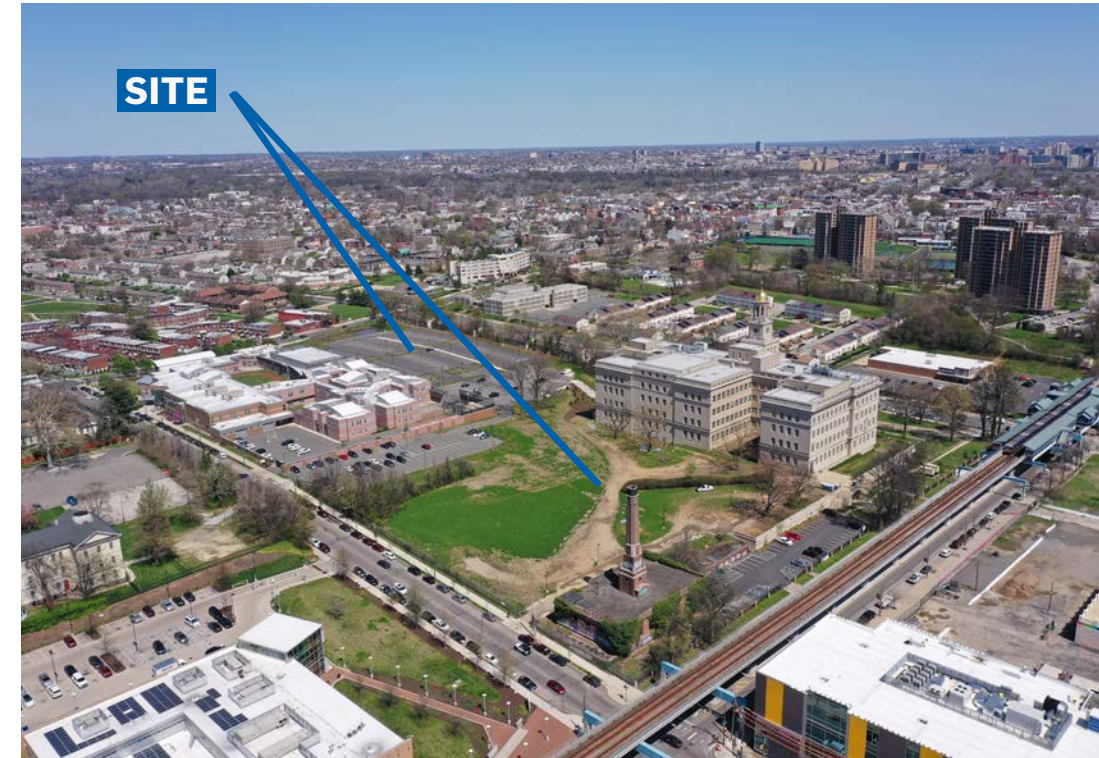
A-4: AERIAL VIEW OF SITE LOOKING NORTHEAST
