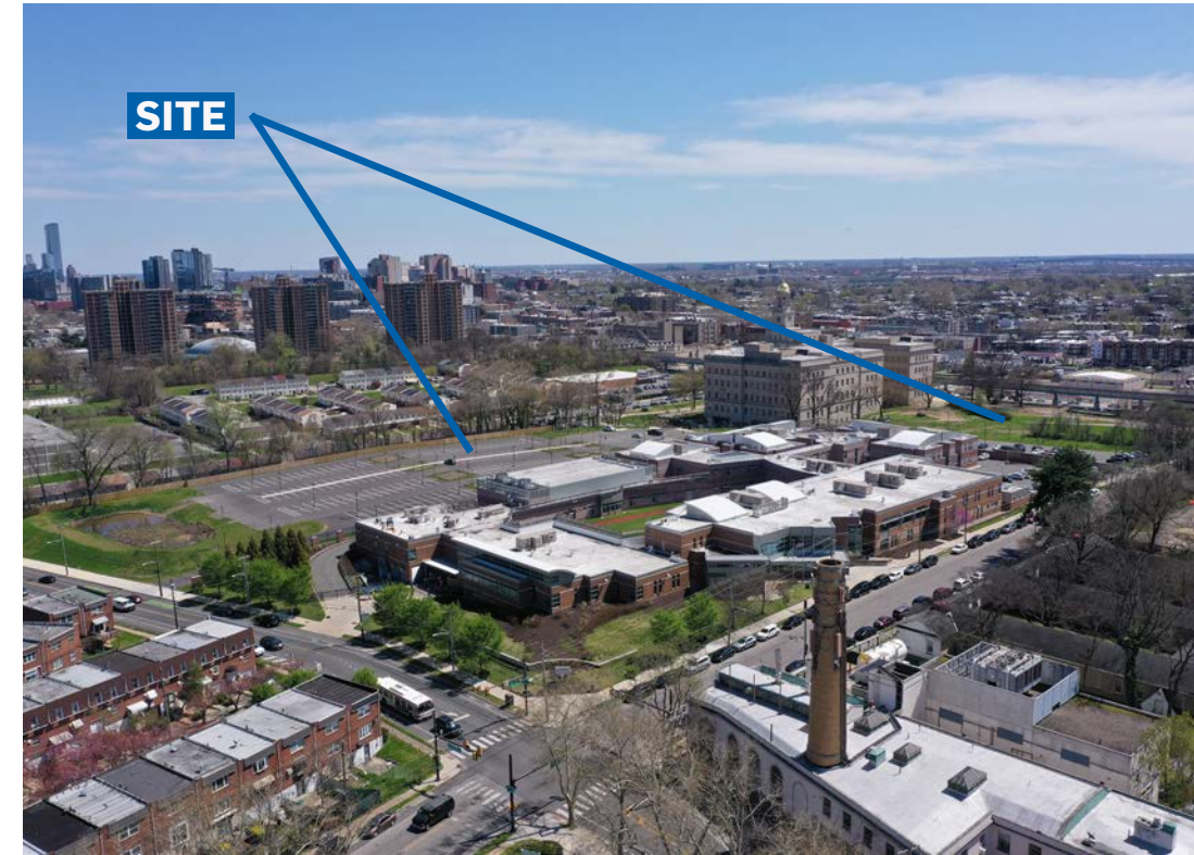
A-6: AERIAL VIEW OF SITE LOOKING SOUTHEAST
