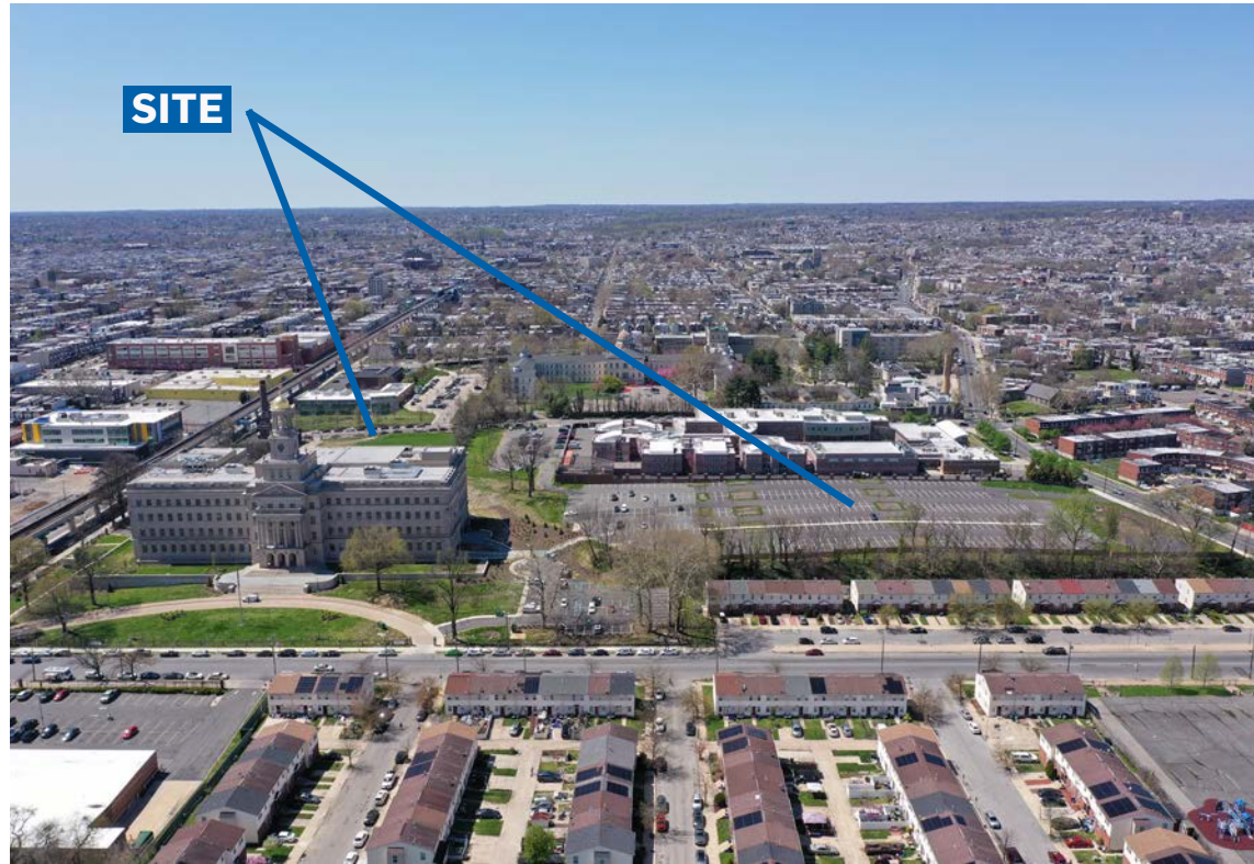
A-1: AERIAL VIEW OF SITE LOOKING WEST
