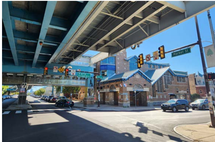
N-2: 46TH & MARKET STREETS CORNER FACING SOUTHEAST
