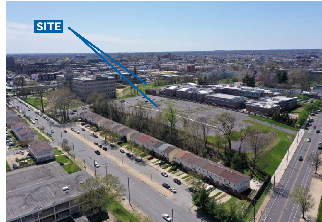
A-8: AERIAL VIEW OF SITE LOOKING SOUTHWEST
