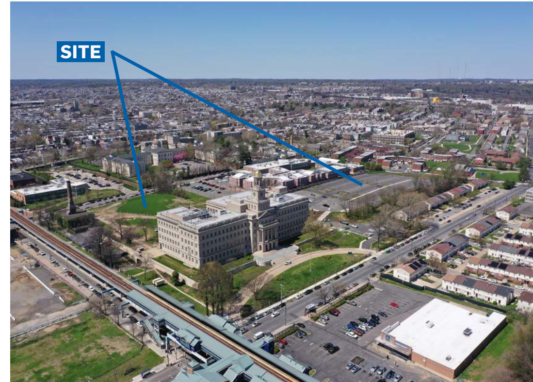
A-2: AERIAL VIEW OF SITE LOOKING NORTHWEST
