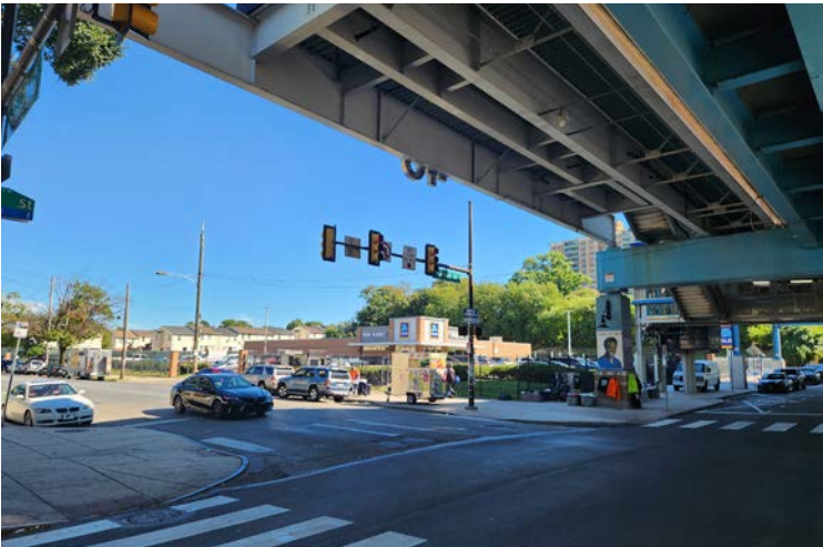
N-1: 46TH & MARKET STREETS CORNER FACING NORTHEAST
