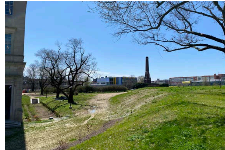
S-11: ON SITE FACING SOUTHWEST TOWARDS MARKET ST
