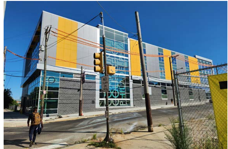
N-4: 48TH & MARKET STREETS CORNER FACING SOUTHEAST
